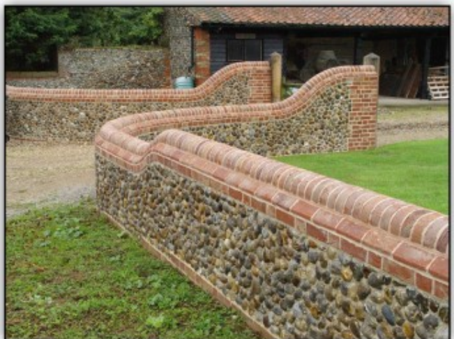
A traditional canted brick and half round coping.
