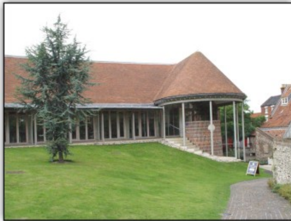
The Shrine of Our Lady of Walsingham - a new refectory building which achieves a high standard of design in a sensitive location.
