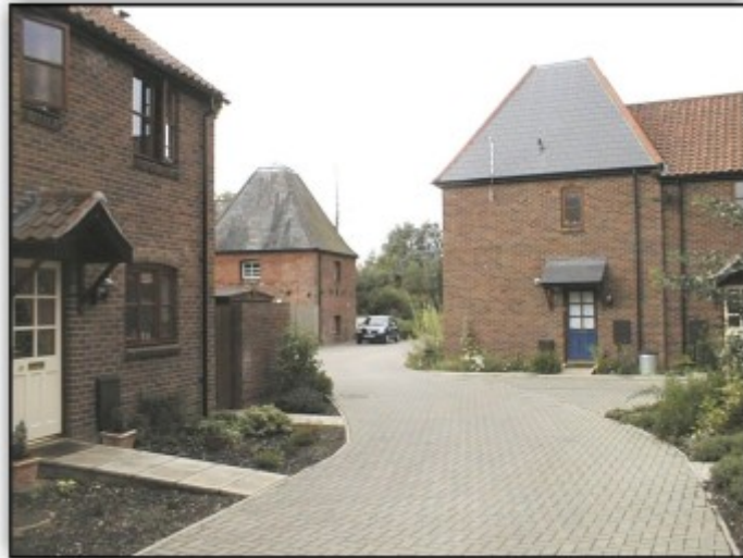
Hall Staithe, Fakenham - a serpentine access road with paved surfacing
