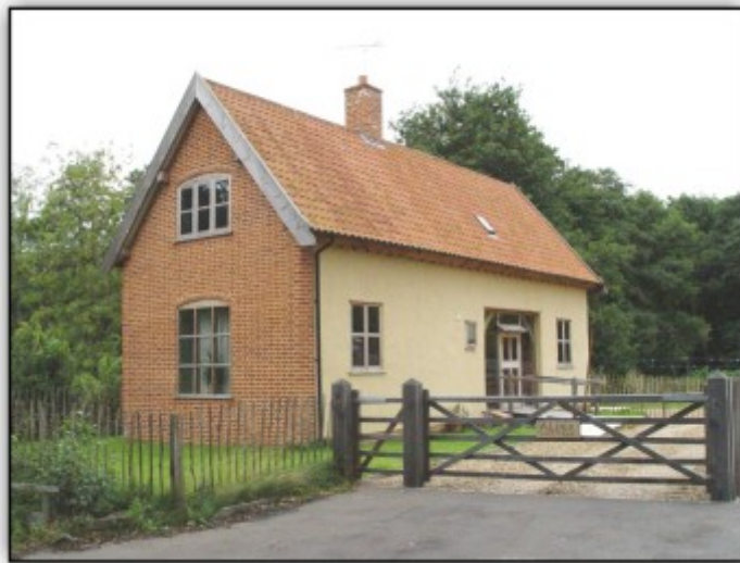
Union Road, Smallburgh - a new low carbon dwelling which has been rendered in lime and finished in limewash.
