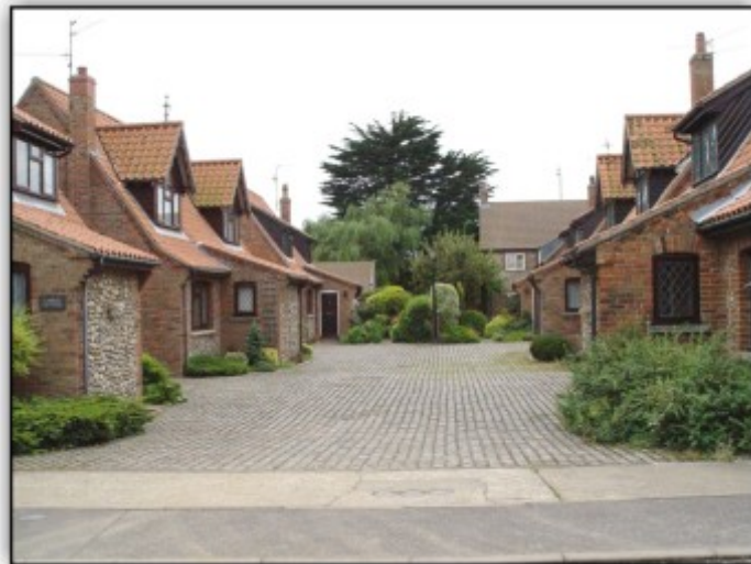
Ramms Court, Wells-next-the-Sea - a shared access surfaced in setts.
