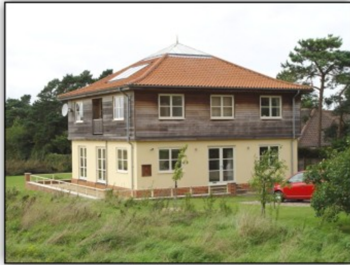
Saxlingham Road, Blakeney - a new dwelling partly constructed in rammed earth.
