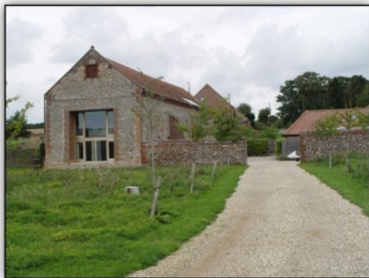
Lower Farm Barns, Barsham - a conversion scheme which reuses existing openings and which mixes historic fabric with contemporary detailing.
