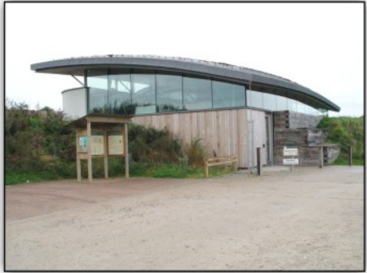
Cley Marshes Visitor Centre - a curved sedum roof allows this contemporary building to respond to its sloping site.
