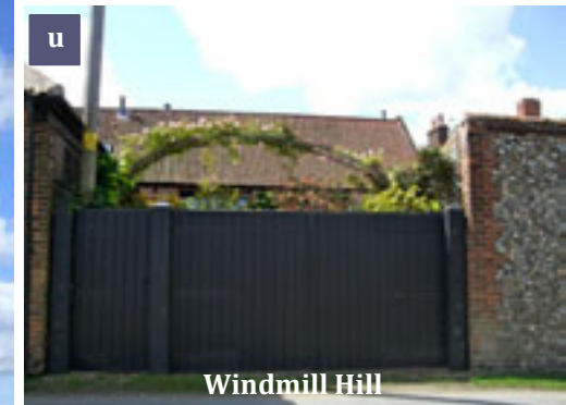
Timber clad outbuilding
