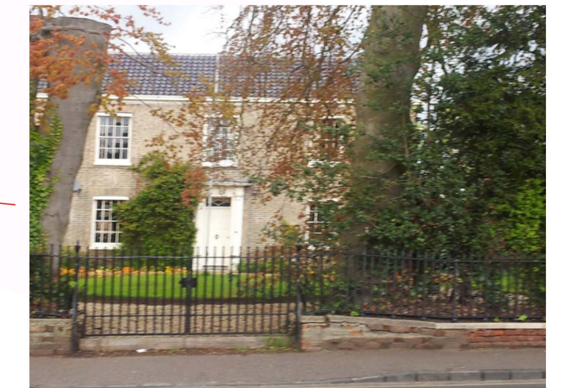
Linstead House - Buff brick, smut pantiles, multi-paned Georgian style windows and doorcases (Yarmouth Road - opposite Heron Gardens west)
