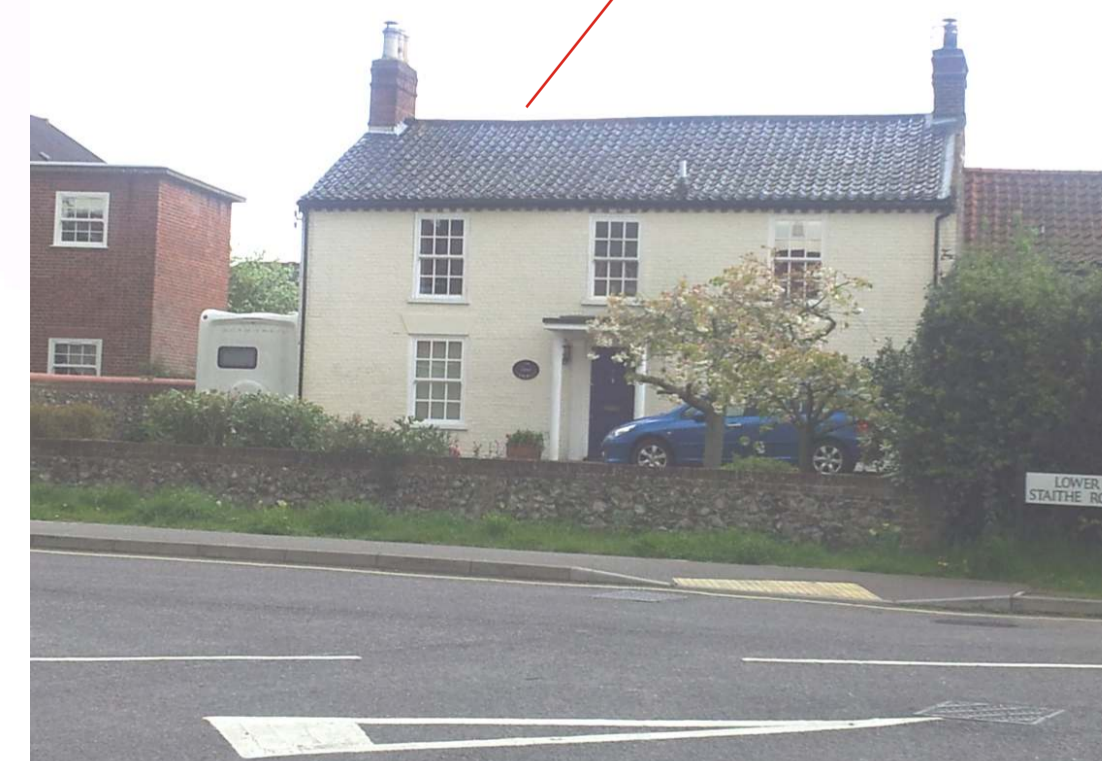
Rendered walls with smut pantiles, simple eaves and verge details, multi-paned sash windows (junction off Old Market Road and Lower Staithe Road). Buildings marking corners of streets / junctions
