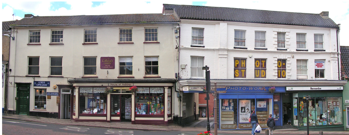
Figure 13 : Kings Arms Street forms the west end of Market Place. A mix of good and indifferent shop fronts.
