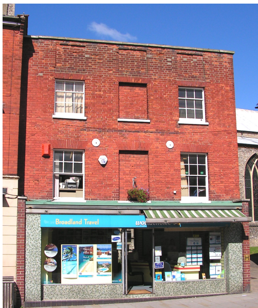
Figure 52 : Plain classical front with parapet hiding the low-pitched roof. The window recesses at the centre may have been introduced for reasons of symmetry, rather than being blocked to avoid paying window tax.
