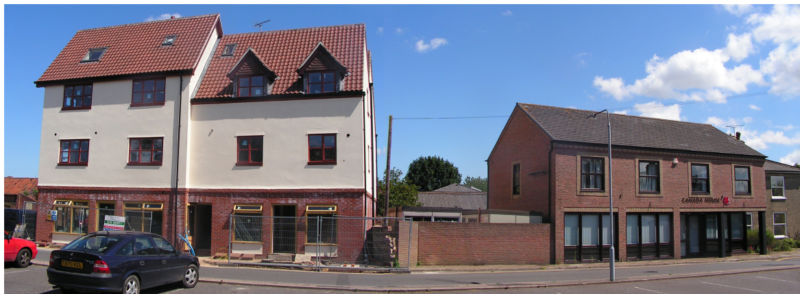
Figure 58 : Poor modern house designs along the south part of Bank Loke
