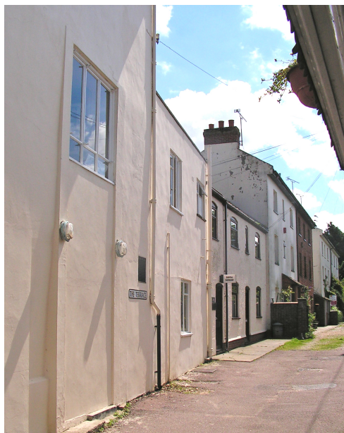
Figure 7 : Historic buildings along the Terrace.
