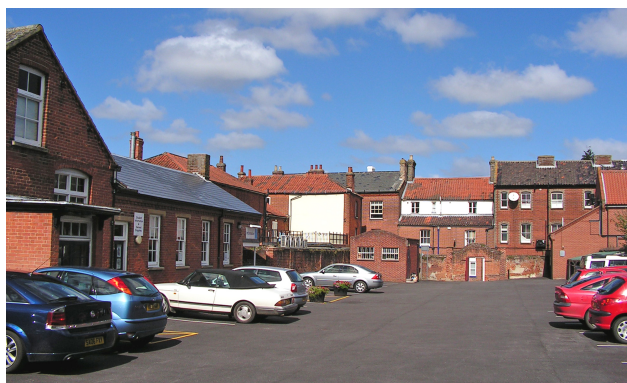
Figure 35 : Courtyard to the north of the Nelson building.
