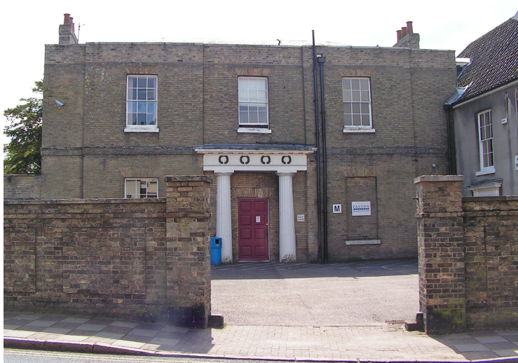
Figure 36 : The Scarborough building viewed from Market St.
