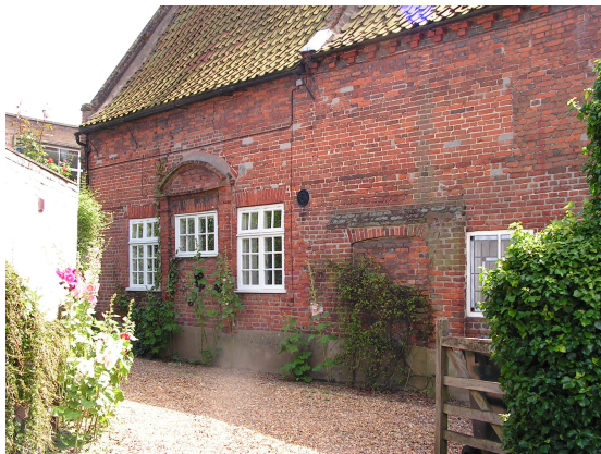
Figure 50 : Ivy Cottage, Aylsham Road. An early 18th century cottage.
