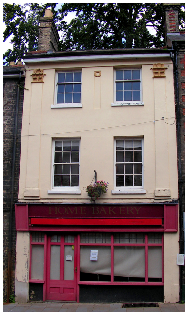
Figure 53 : 44 Market Place: Stucco-work with moulded pilasters.
