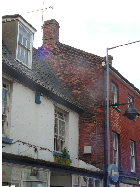
Figure 49 : 3 Market Place. A refronted house where the roof pitch has been changed.
