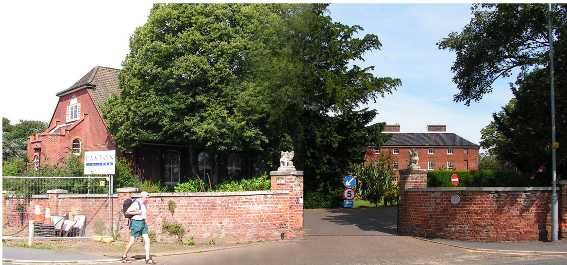
Figure 33 : Main entrance to Paston College.
