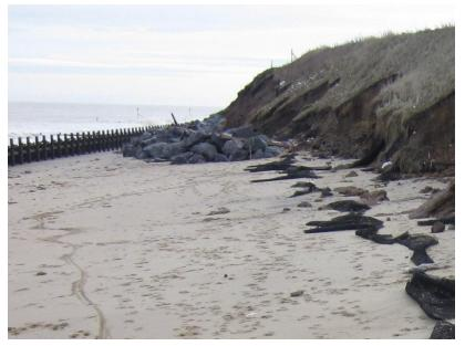
*Figure 4. Cliff erosion behind rock revetment at Bacton* **Bacton following the December 2013 storm surge event.**
