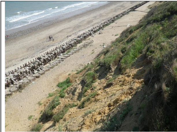
Boulder-fill baskets protecting the cliff toe at Trafalgar Court access
