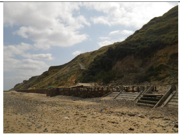
Overview of the northern section of the site showing transition from boulder-filled gabions to detached palisade fence
