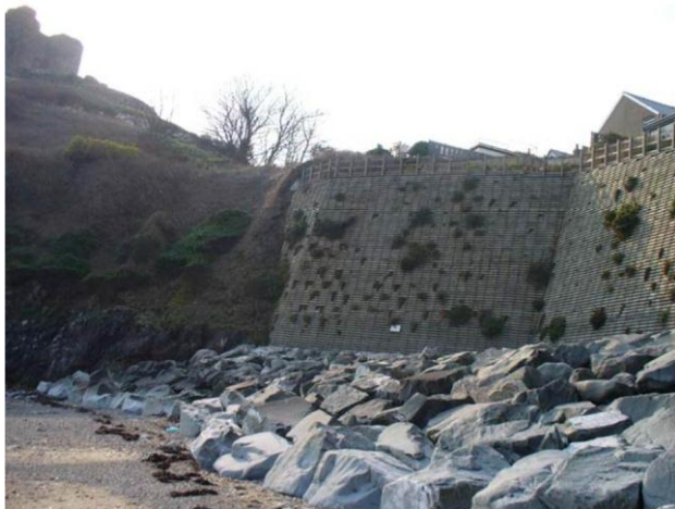
Example of a crib-lock wall
