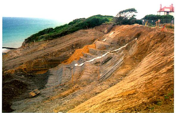
Figure 8 - Benching of Earthworks and Installation of Under Drainage
