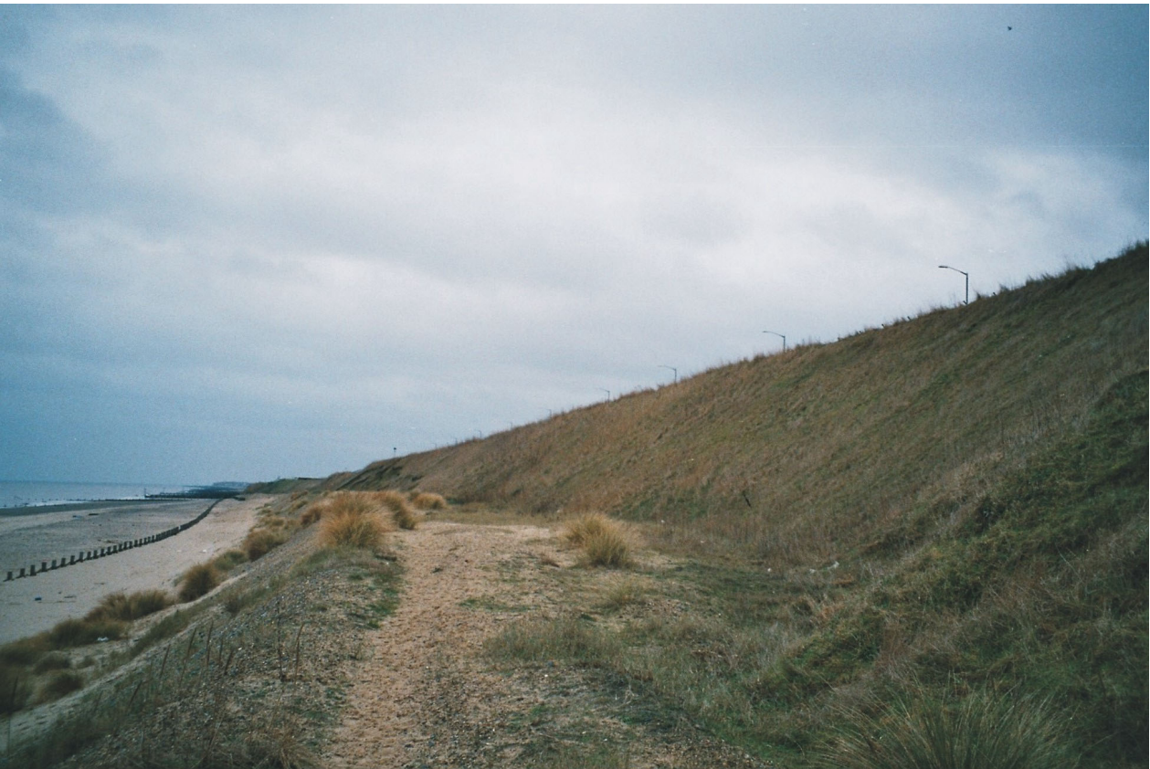
Plate 4 Cliff behavioural unit 18 – view east; note the regraded slopes
