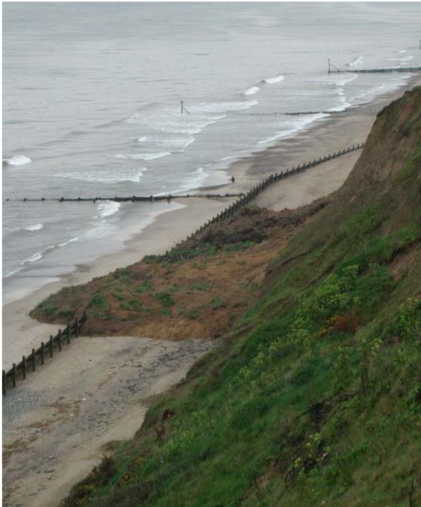
Figure 4 Undercutting and erosion induced cliff failure
