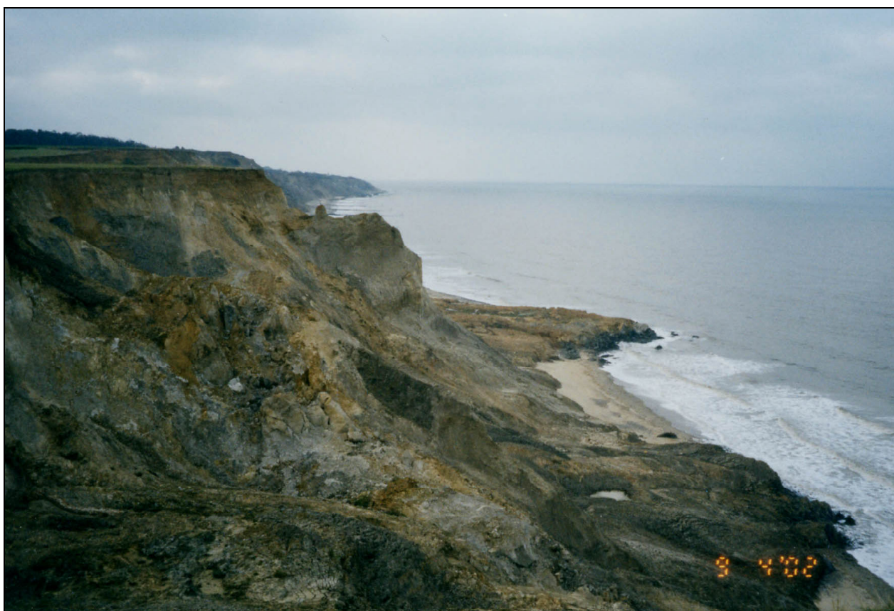
Figure 5.1 Landsliding on the coast, west of Trimmingham (view westward)
