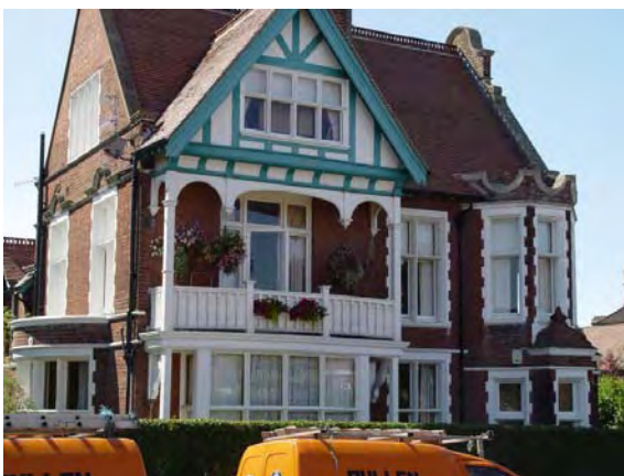
Balcony at 4 Cliff Avenue
