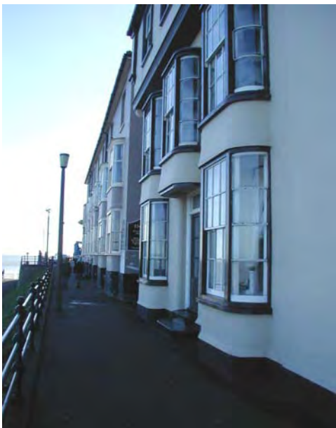
Examples of bay windows at West Cliff
