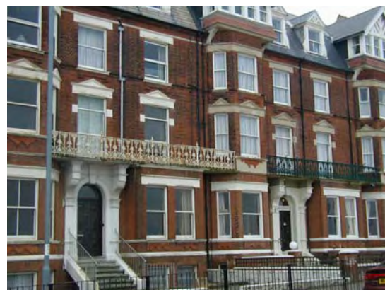
Balcony at Anglia Court, Runton Road
