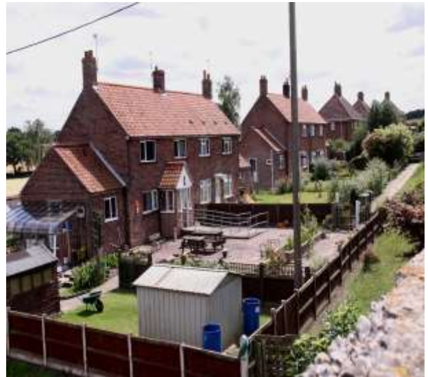
12 Council Housing on Heydon Road
