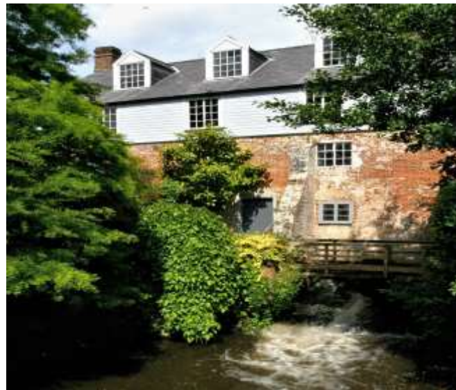
8 The mill showing wooden cladding, brick with classical dormer windows
