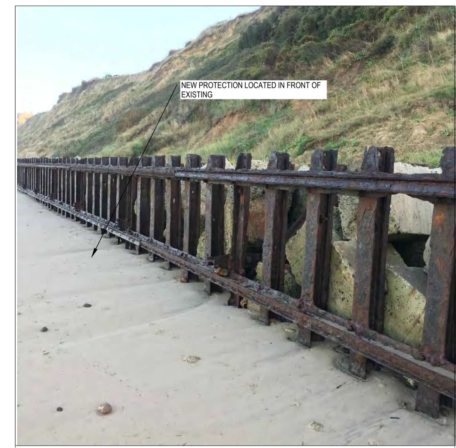
PHOTOGRAPH OF EXISTING STEEL FRAMED DEFENCE
