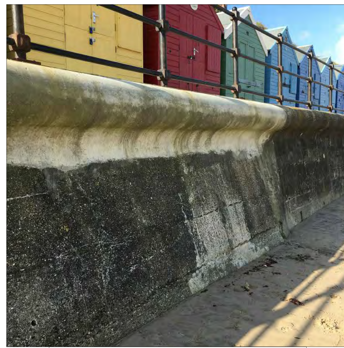
PHOTOGRAPH OF EMERGENCY REPAIR TO SEAWALL AT SEAWALL FRONTAGE 2A
