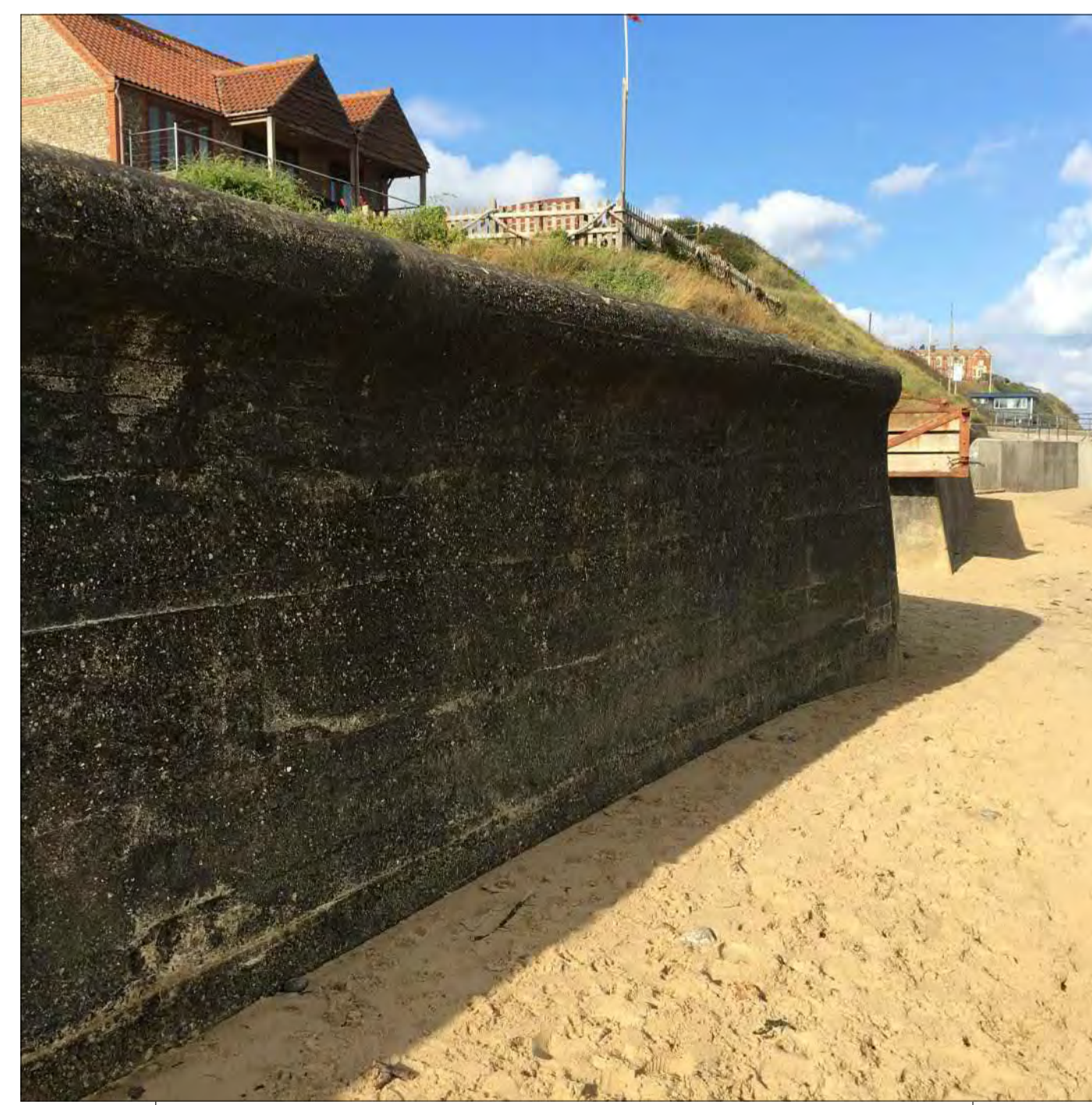
PHOTOGRAPH OF CURRENT SEAWALL AT SEAWALL FRONTAGE 5
