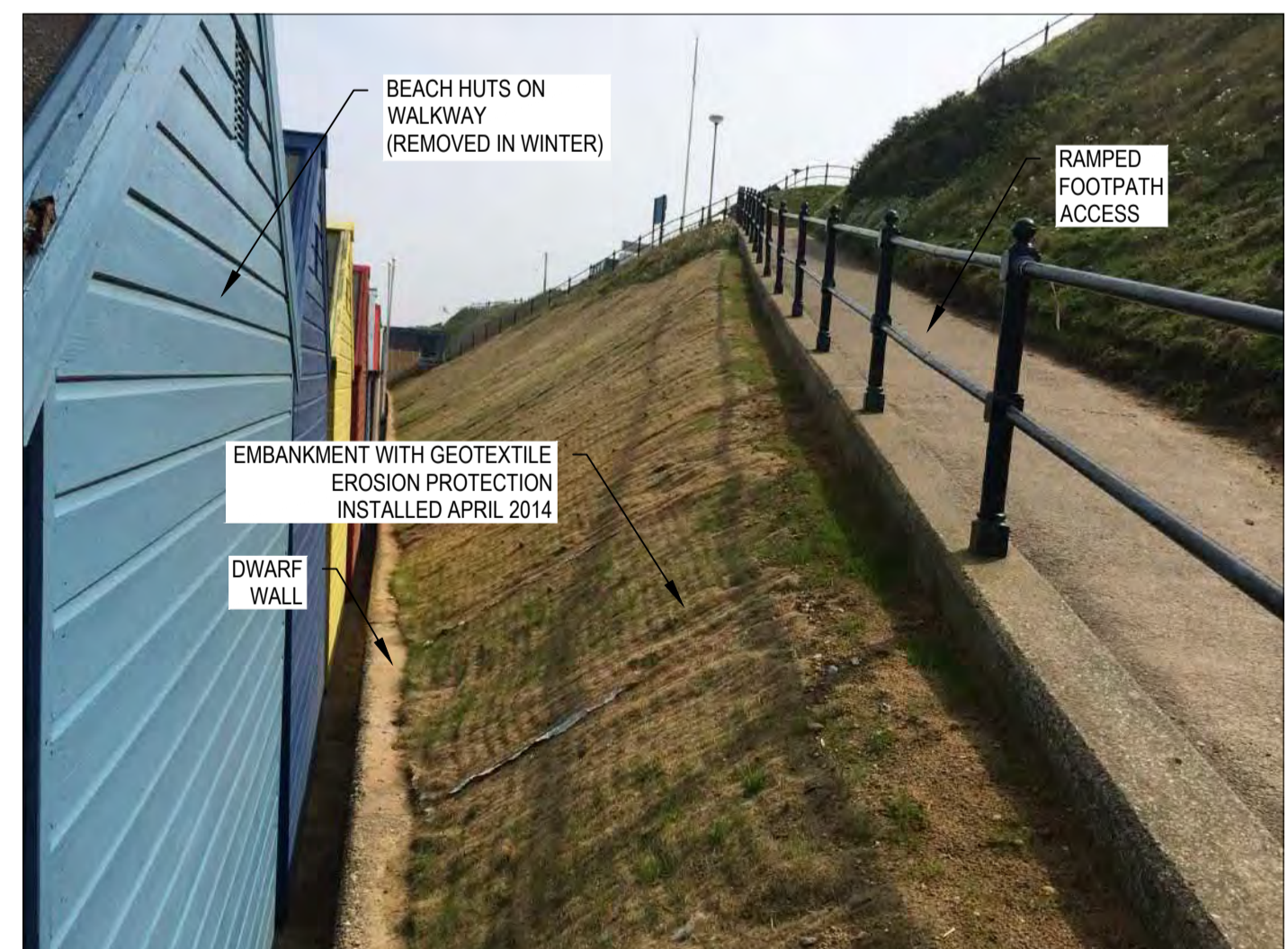
PHOTOGRAPH OF EXISTING EMBANKMENT (NOTE EXISTING GEOTEXTILE EROSION PROTECTION UNDERTAKEN IN 2014)
