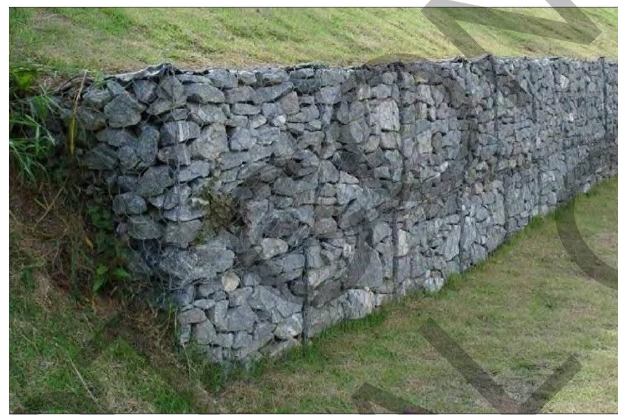
EXAMPLE OF GABION SCOUR PROTECTION
