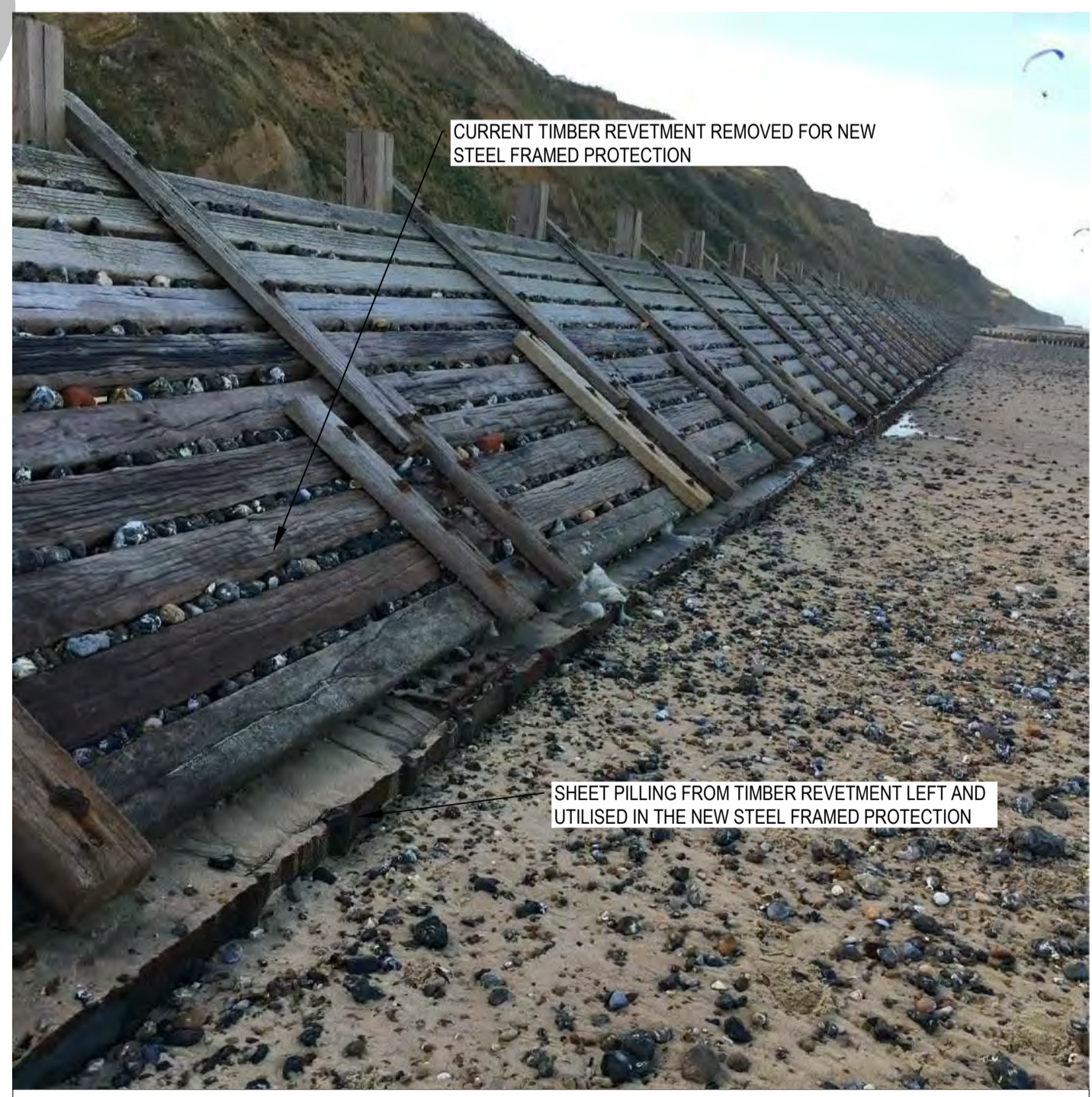
PHOTOGRAPH OF EXISTING TIMBER REVETMENT
