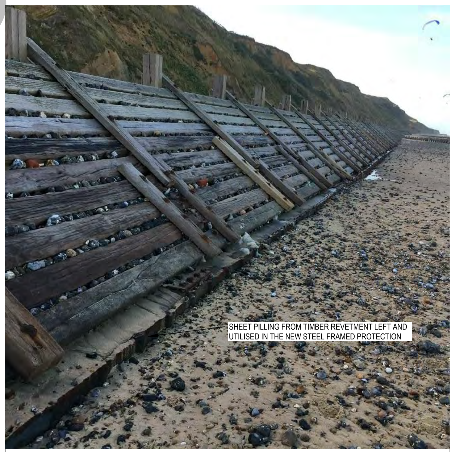
PHOTOGRAPH OF EXISTING TIMBER REVETMENT
