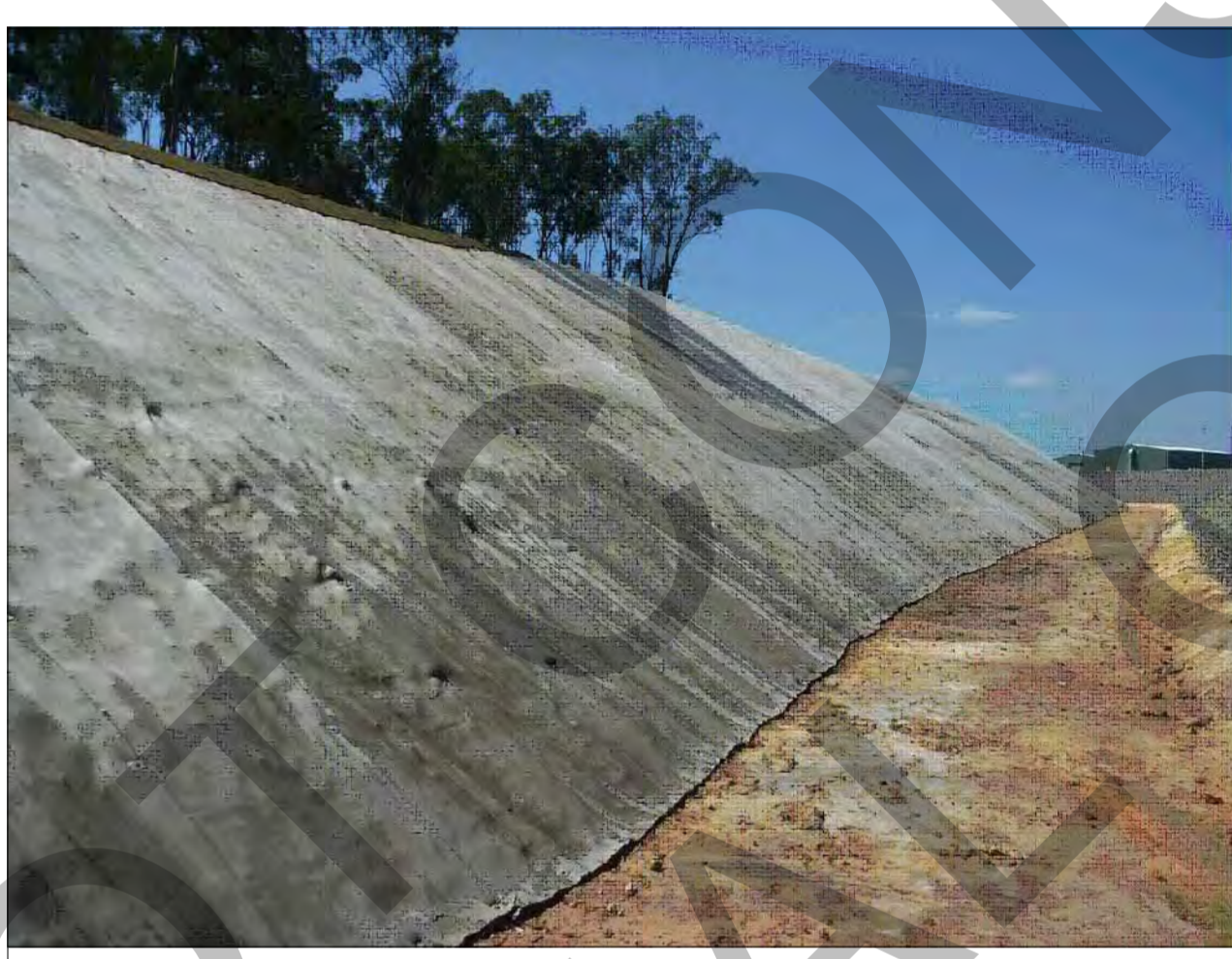
EXAMPLE OF SPRAYED CONCRETE SCOUR PROTECTION PHOTOGRAPH COURTESY OF BURDENS
