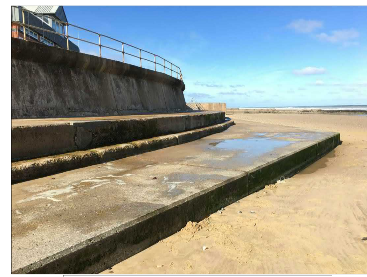
PHOTOGRAPH OF CURRENT SEAWALL AND APRON AT SEAWALL FRONTAGE 6
