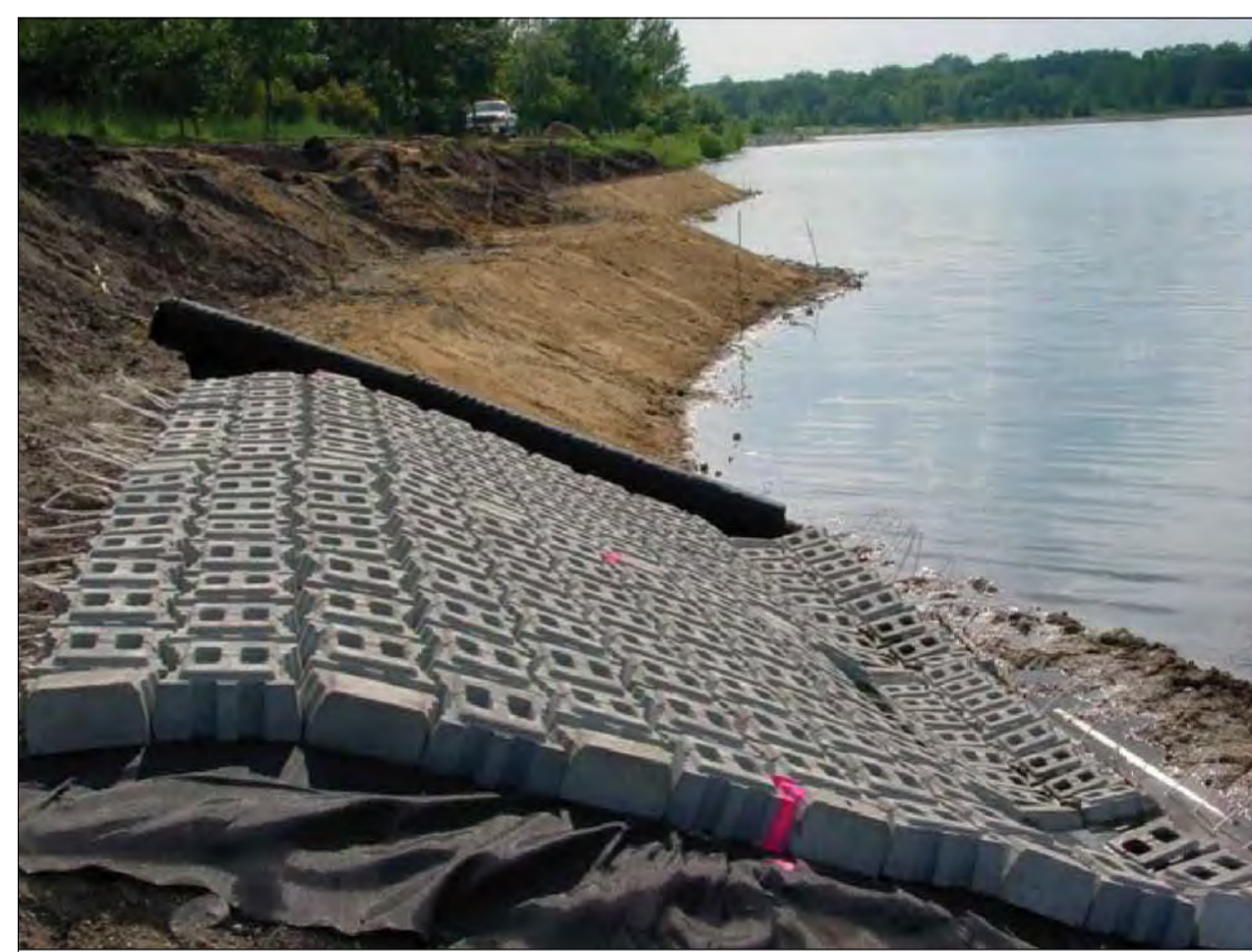
EXAMPLE OF CONCRETE BLOCK SCOUR PROTECTION PHOTOGRAPH COURTESY OF CONTECH ENGINEERED SOLUTIONS
