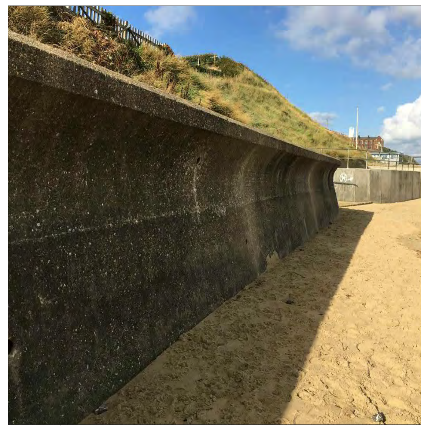
PHOTOGRAPH OF CURRENT SEAWALL AT SEAWALL FRONTAGE 4
