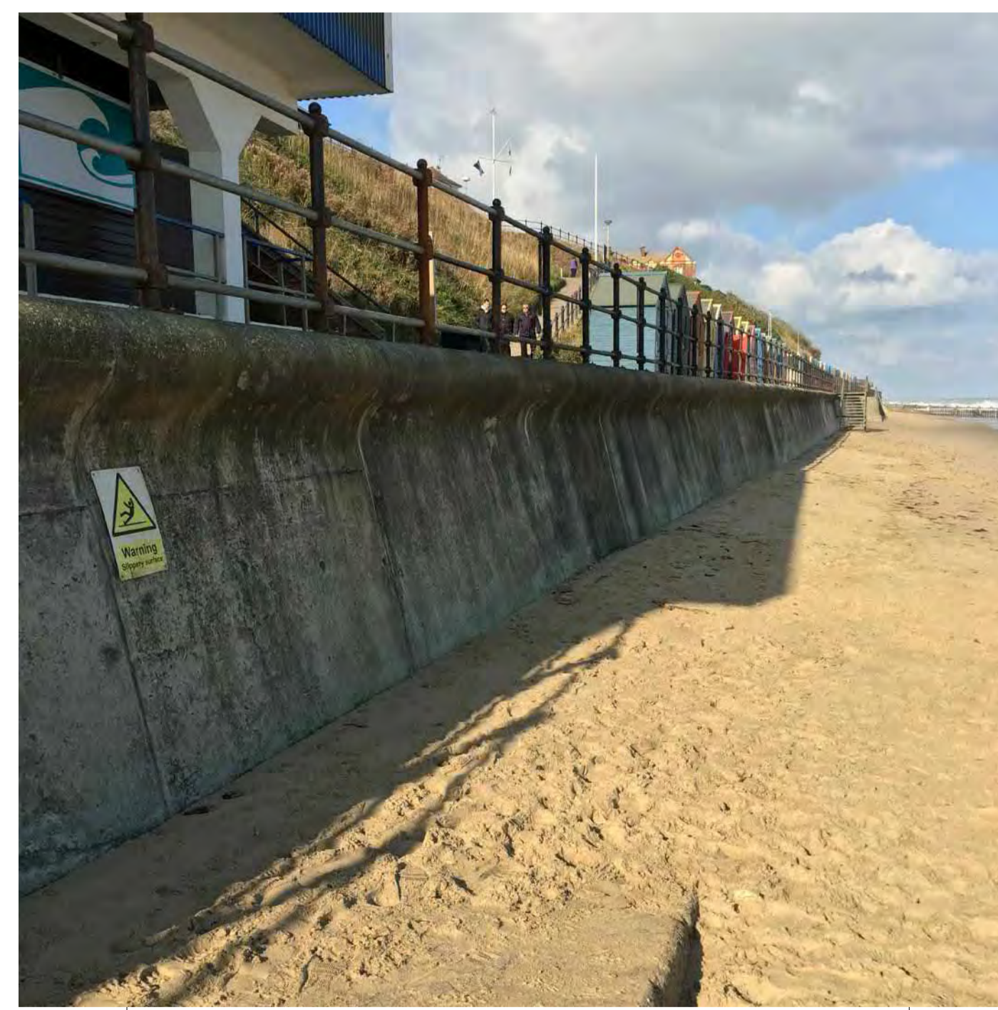
PHOTOGRAPH OF CONCRETE SEA WALL AT SEAWALL FRONTAGE 2B
