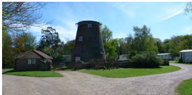
The former mill within the caravan site
