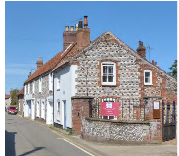
Brick and flint used in decorative patterns on a house on the High Street
