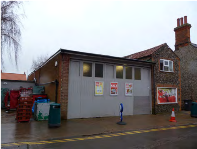
Garish advertisements on the Spar storage unit, with unattractive crates and other items stored adjacent
