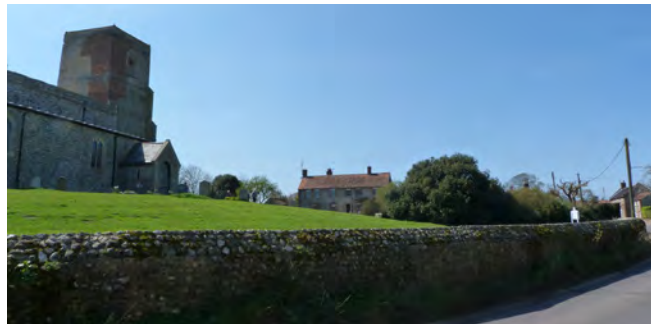
Flint boundary wall to the churchyard
