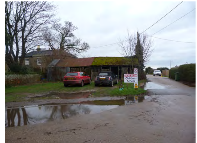
Dilapidated sheds to the north of the Green, with ad-hoc signage at the entrance to Quay Lane
