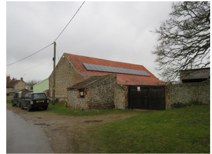
Solar panels on Church Farm barn
