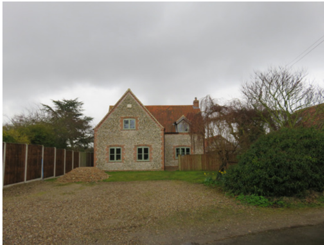
Loss of a sense of a defined boundary in front of the new house on The Street
