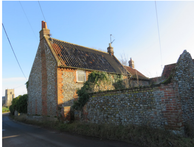
Green Farmhouse and shed, Blakeney Road
