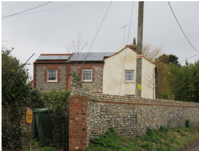
Solar panels on Sunny Corner are made more prominent by the rise in the land
