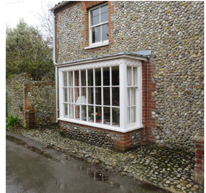
Cobbled floorscape on Chapel Lane is being damaged by vehicles
