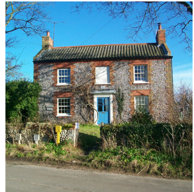
Detached historic brick and flint house, Sycamore House, The Street
