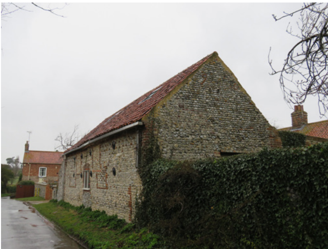
Converted barn of Primrose Farm, Chapel Lane
