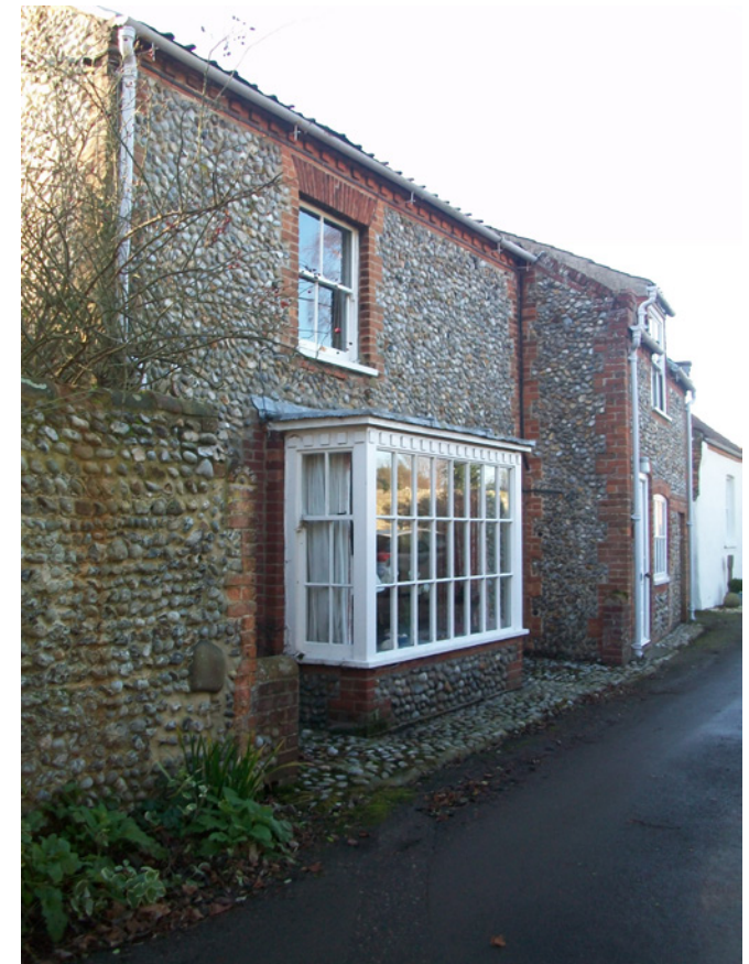
Possible historic shop front on Chapel Lane
