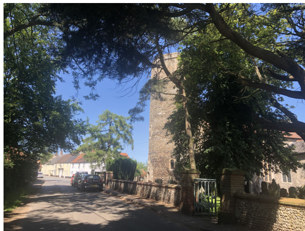
Picture 6 St Andrews Church & Cottages, Station Road (July 2019)
