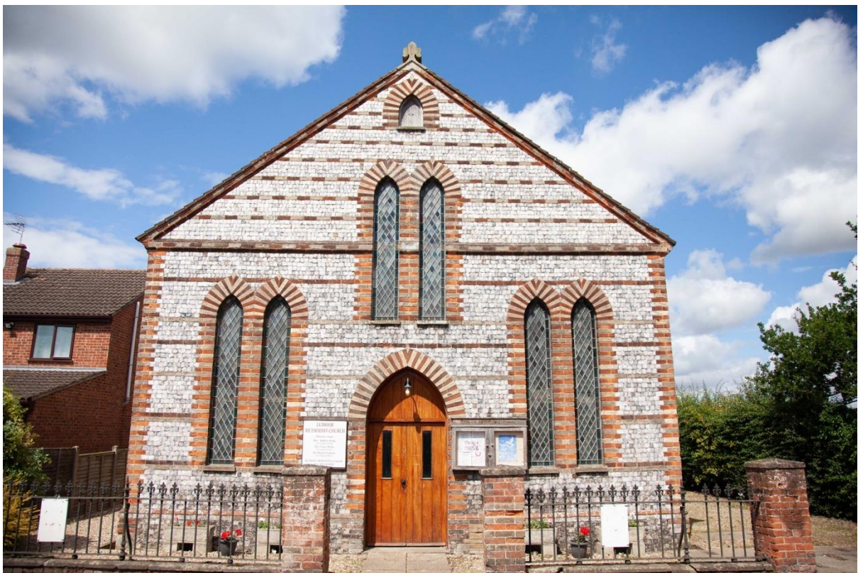
The Methodist Church faced with its fine knapped flintwork
