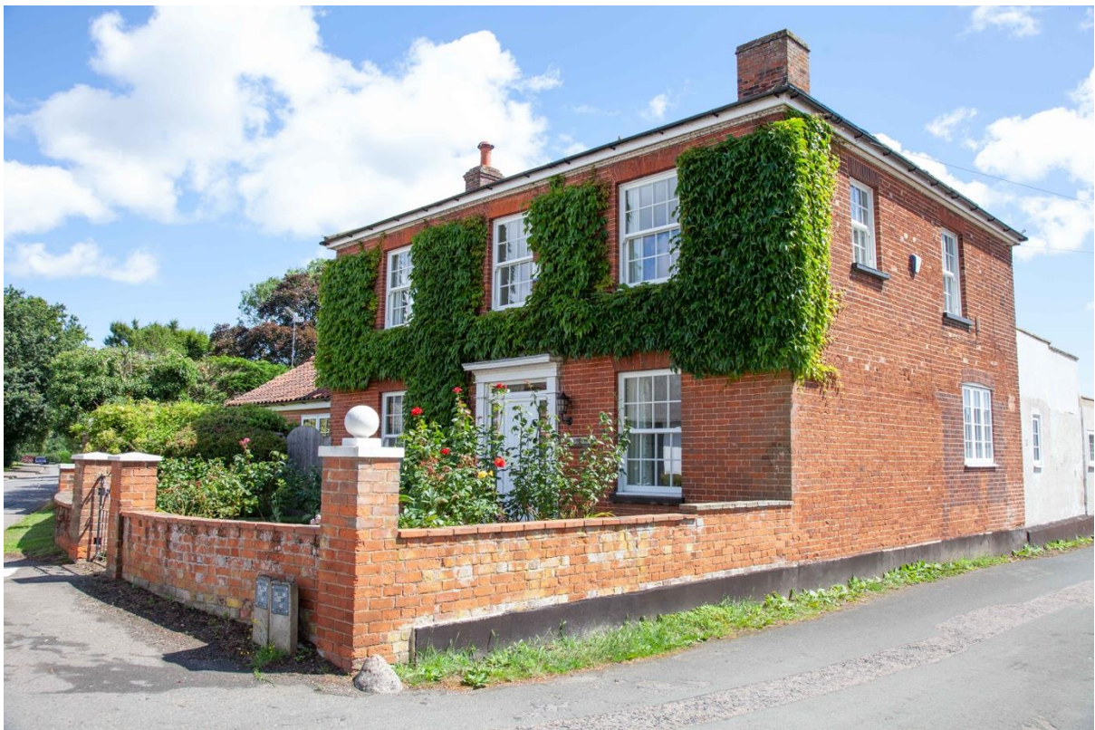
Albury House on the corner of Malthouse Lane contributes to the character of the area
