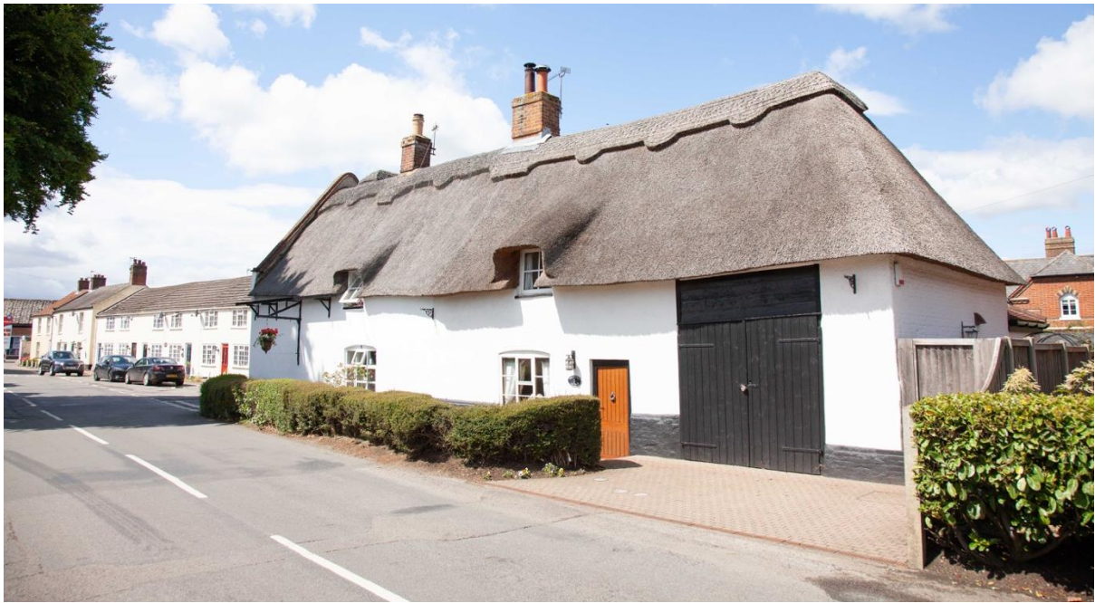
The Stores is a listed building dating from the early 18th century
