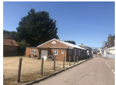
Picture 3 Great Ryburgh Memorial Hall, Built 1952 (July 2019)
