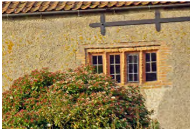
Brick mullioned window on the farmhouse at Pitt Farm which stylistically dates to the 16th or 17th century
