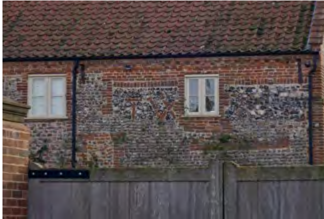
Dales House, with interesting brickwork patterns spelling out 'TW'
