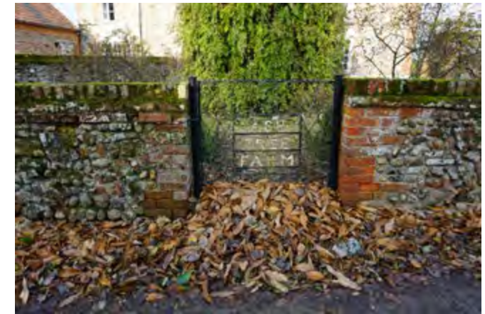
Brick and Flint wall with decorative metal gate to Ash Tree Farm
