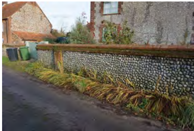
Low brick and flint wall on The Street
