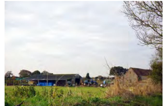
Modern barn seen from The Street
