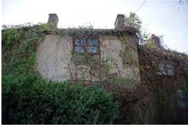
Cementitious render repairs
