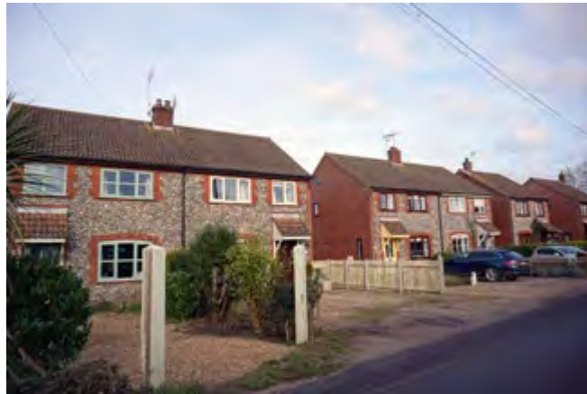
Flint and brick late-twentieth century semi-detached cottages on The Street
