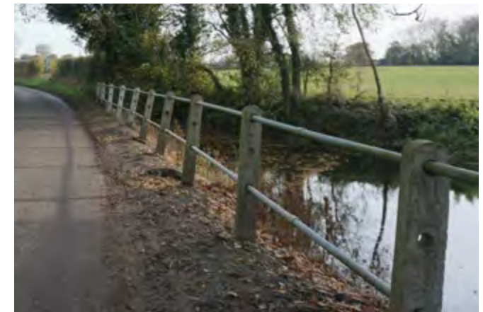
Concrete post and steel pole fence, which is not in keeping with the character of the village
