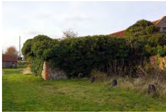
Remains of a barn at Manor Farm House
