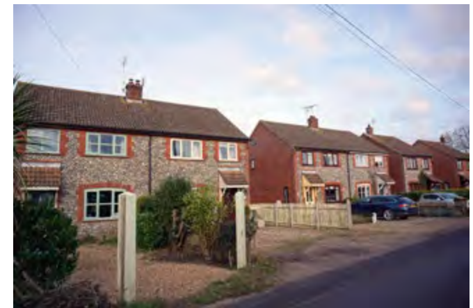
Front gardens converted to driveways
