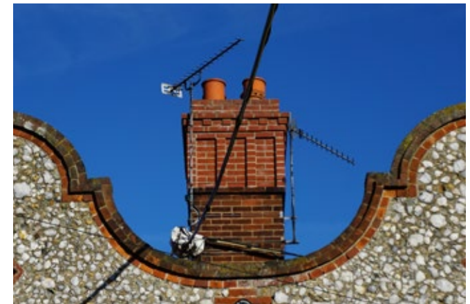
Aerials and wiring clutter the appearance of facades
