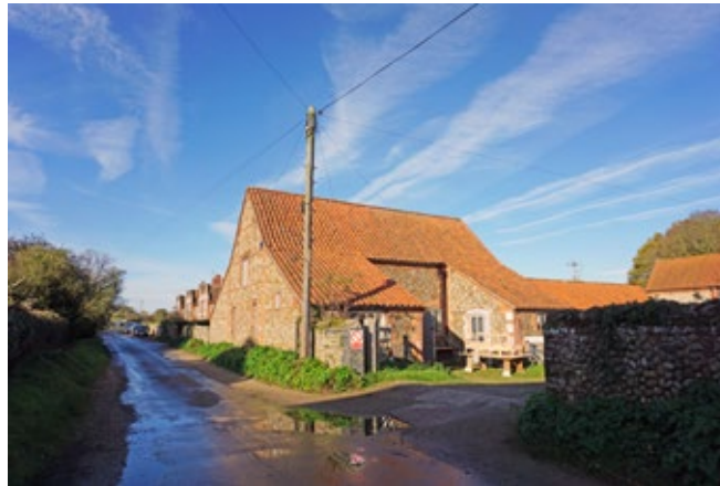
Barn with catslide roof, converted to light industrial use
