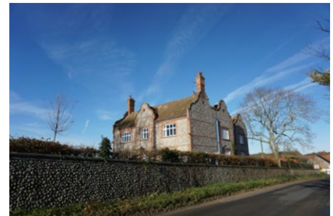
Long flint wall demarcating the Manor Farm site
