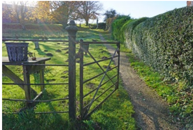
Historic metal gate and fence to the Shell Museum garden
