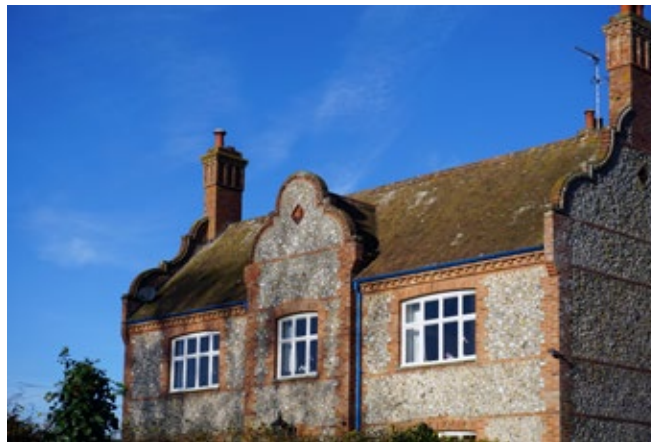
Manor Farmhouse, also featuring the same Dutch gables and use of red brick dressings to flint walls
