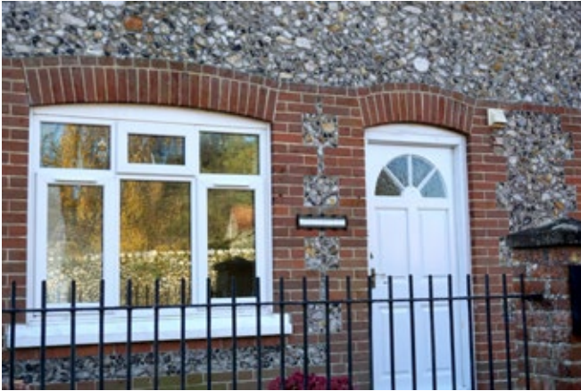
uPVC window and modern replacement door
