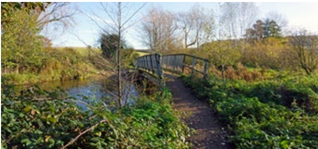
The bridge over the ford
