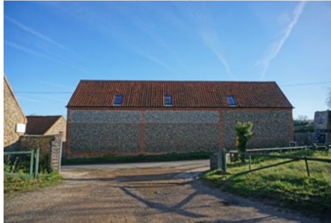
Barn converted to residential use with conservation rooflights inserted
