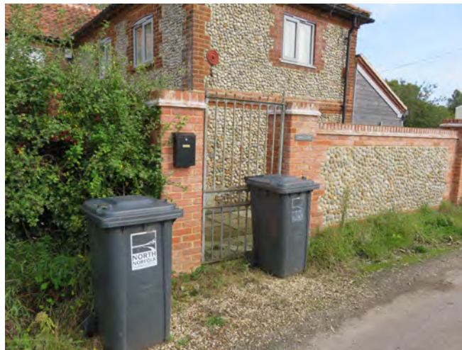
Out of scale new gate piers and wall with letterbox
