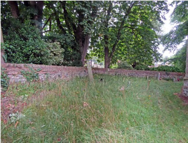
Cobble flint and red brick wall enclosing the churchyard with mature trees and shrubs beyond
