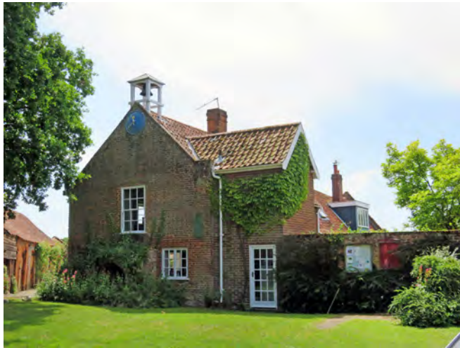
Eighteenth century school building on the Village Green
