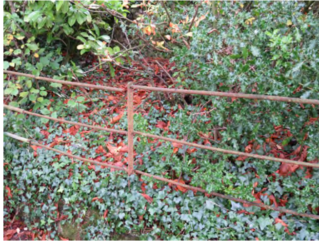
Metal railing to the churchyard
