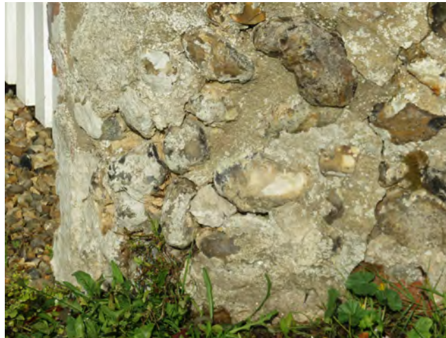
Cementitious pointing to a flint wall
