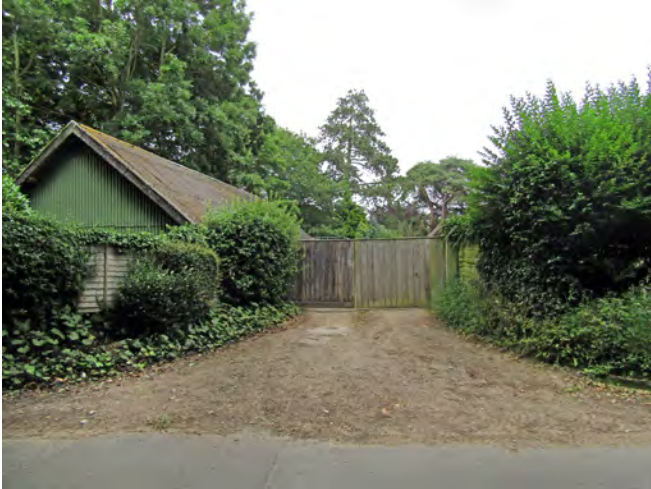
A short stretch of timber fence on the west boundary to Brinton Hall
