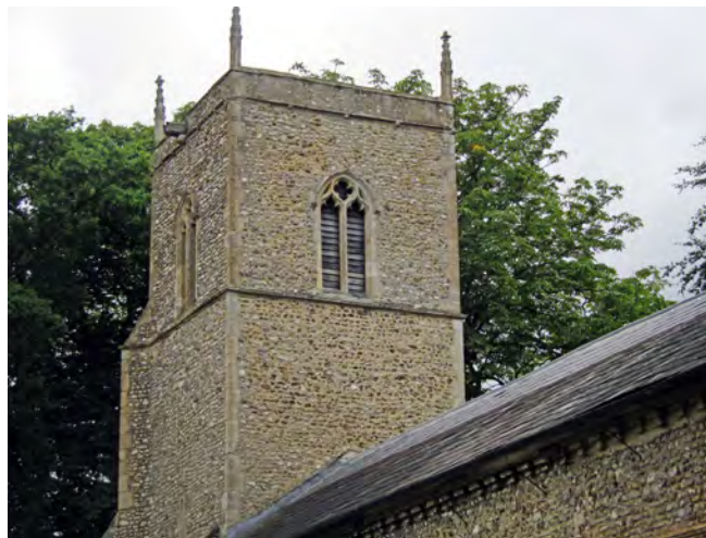
Detailed view of the church tower
