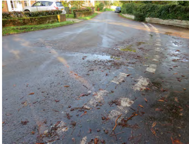
Patched road surface
