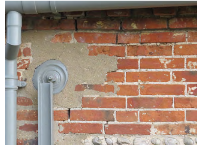
Cementitious repointing to brickwork
