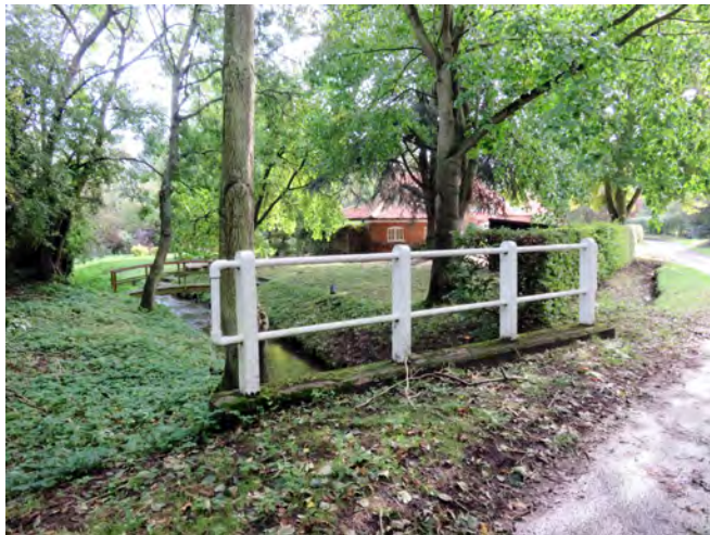
Bridge railing separating public right of way from tributary of the River Glaven
