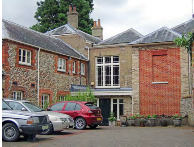
View of the west elevation of Brinton Hall
