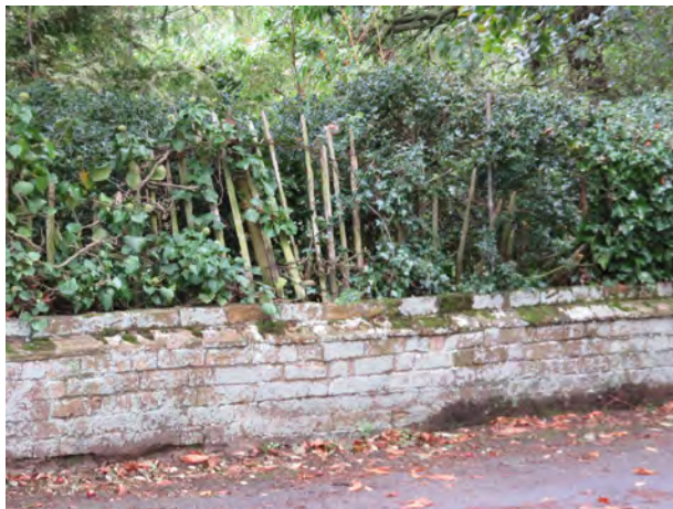
Post and wire replacement fence
