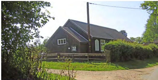
View of the Village Hall from King Street
