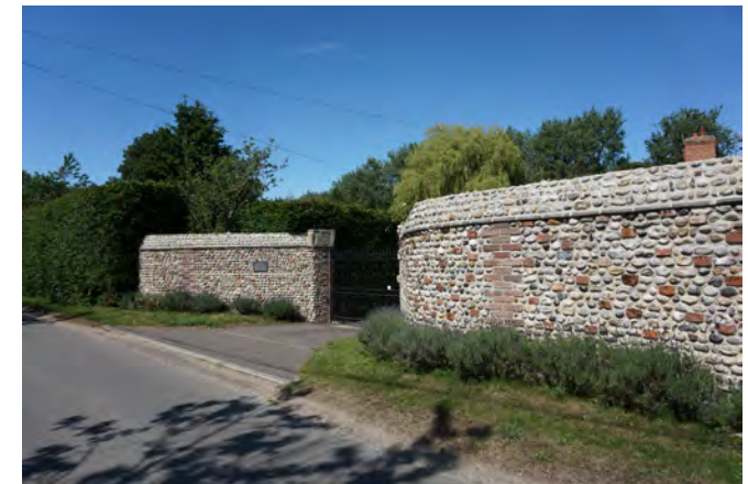
New walls and gate at Green Farm
