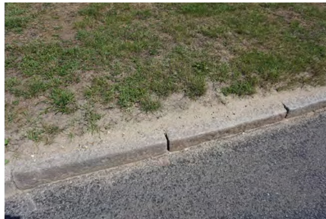
Granite kerb stones on Holt Road
