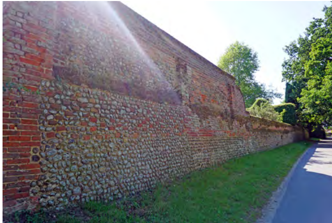
Boundary wall to Hunworth Hall
