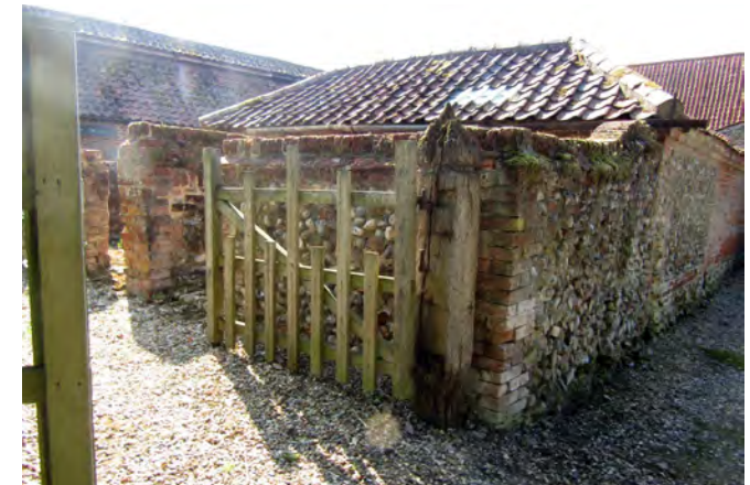
Former pigsties at Hunworth Hall Farm
