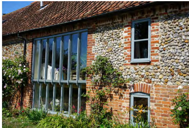
A sensitive barn conversion on King Street
