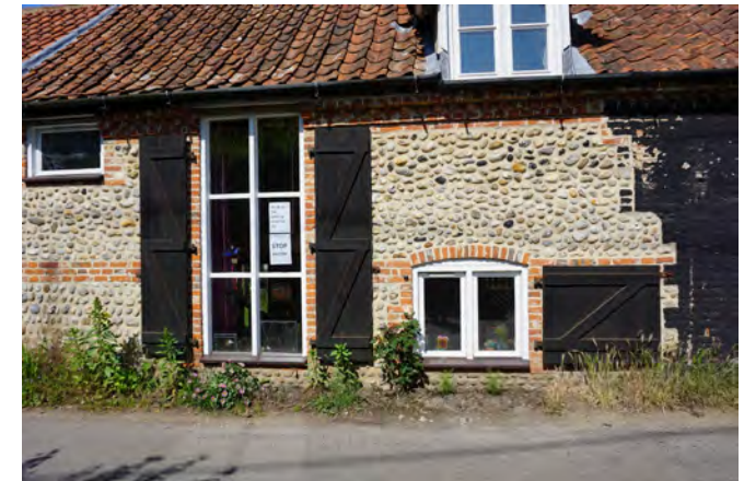
Wooden shutters flanking openings on a barn conversion
