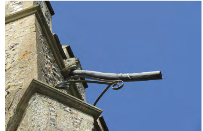
Detail of a gargoyle on west tower
