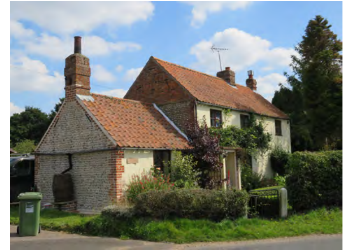
Crossways located situated on Norwich Road
