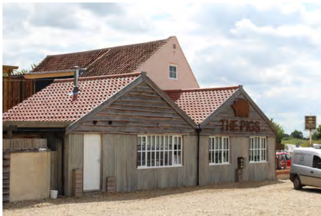
West elevation of The Pigs with date stone located inscribed with '1763' located in the apex of the roof. The single storey elements are recent extensions
