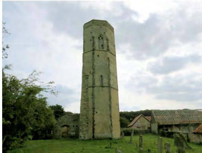
Old Church tower
