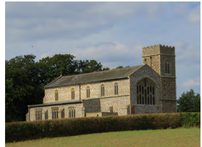
South and east elevations
