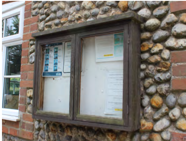
Timber noticeboard located on the Village Hall
