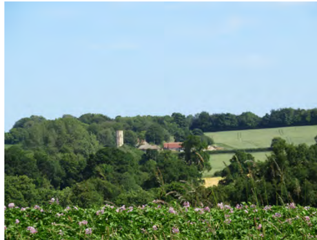
Tower of former Church of St Peter and St Paul situated amongst areas of wood and open fields viewed from Hunworth
