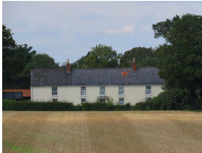
Front elevation of Manor Farmhouse
