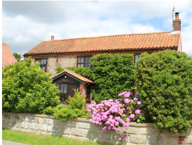
Fourways located on the east-west stretch of Pecks Lane outside the Conservation Area
