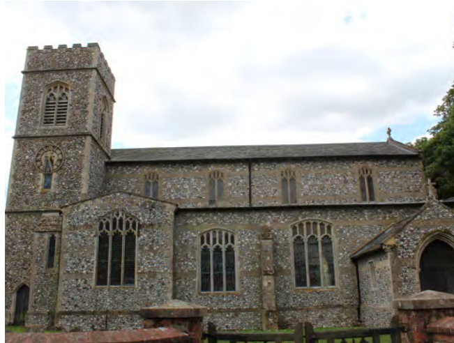
North elevation of the church
