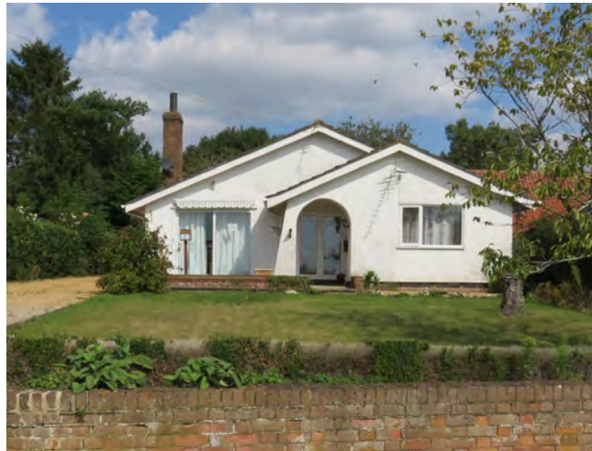
Twentieth century bungalow situated on the north-south stretch of Pecks Lane outside of the Conservation Area
