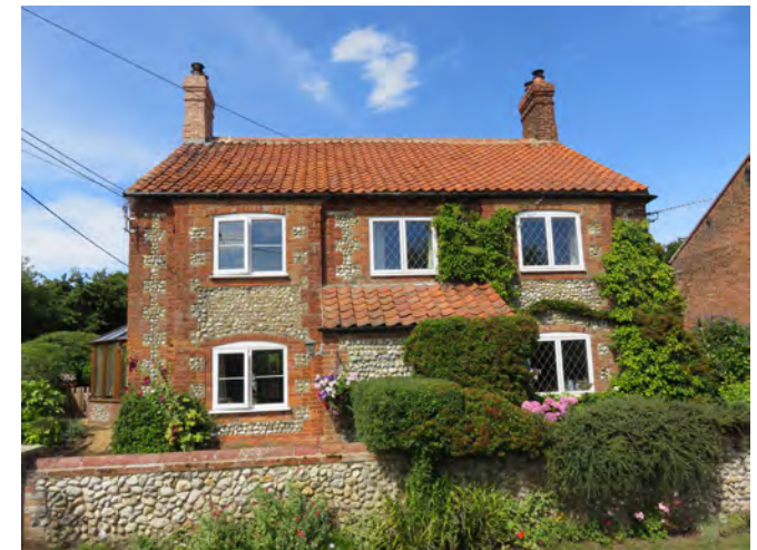
Front elevation of 22-23 Bale Road
