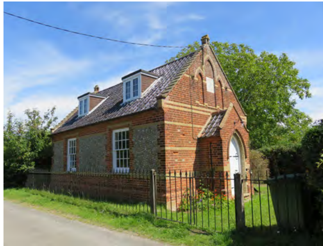
North and west elevation of converted Wesleyan Chapel
