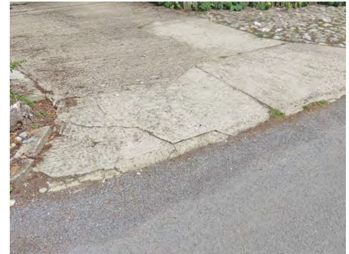
Large concrete splay
