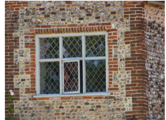
Detail of mullion and transom windows on Sharrington Hall
