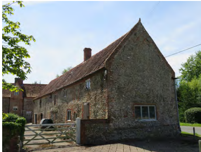
Boundary walls enclosing Sharrington Hall and adjacent farm buildings
