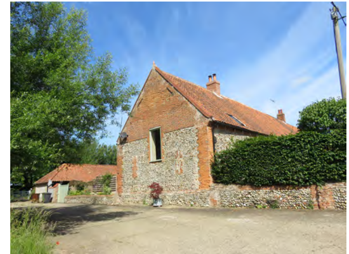
South elevation showing glazed door opening of the Hayloft at the north end of Lower Hall Lane
