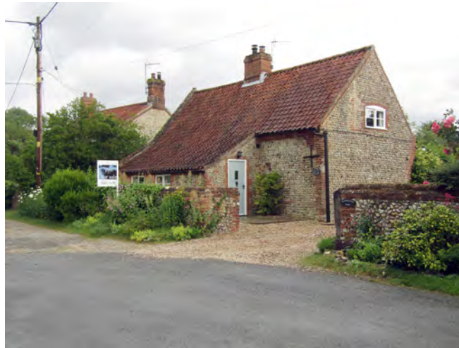
Medium sized historic house located on The Street
