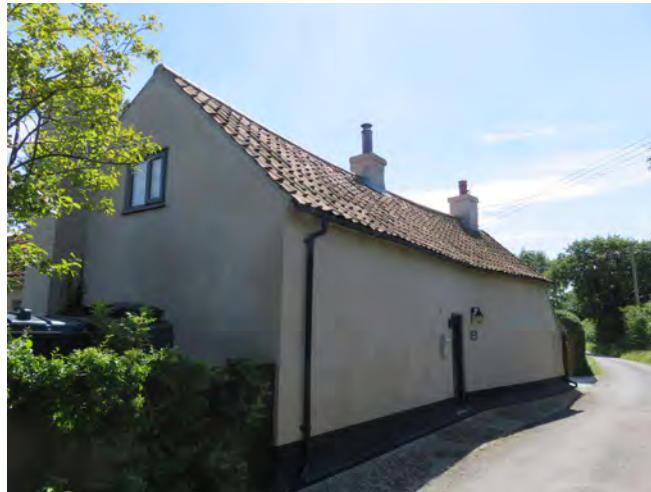
Front rendered elevation of Stone Cottage on the Street
