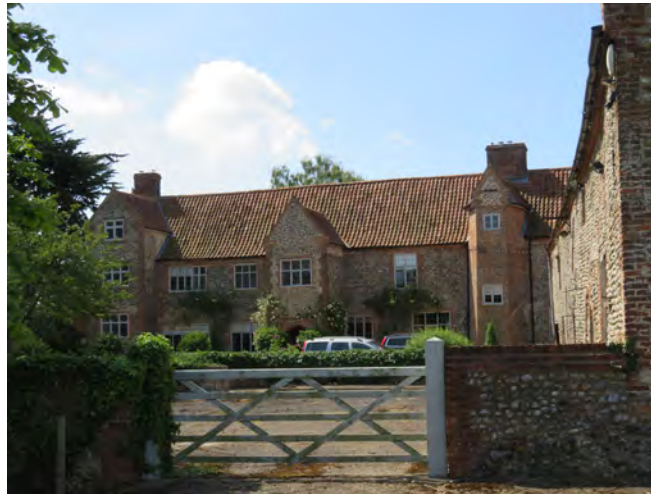
Front elevation of Sharrington Hall
