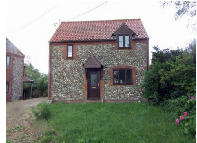
Modern house located on The Street
