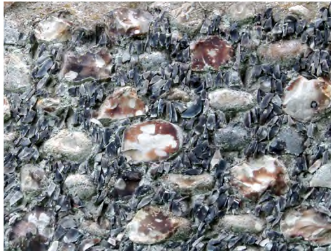
Flint galletting on Sharrington Hall Barn
