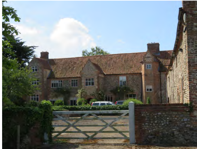
Front elevation of Sharrington Hall
