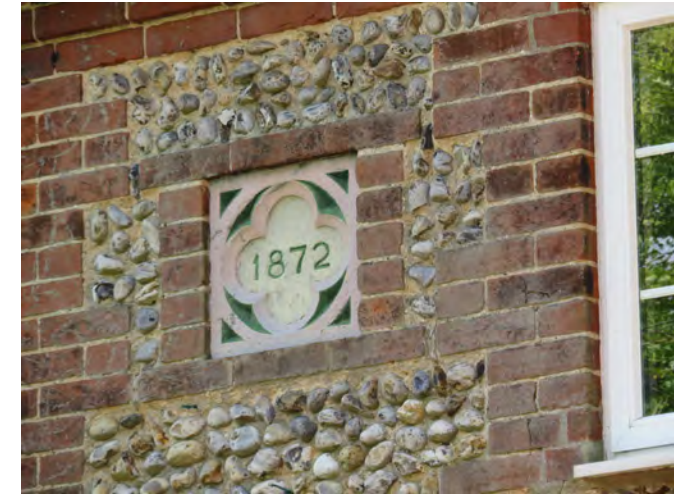
Date stone in quatrefoil surround in terracotta
