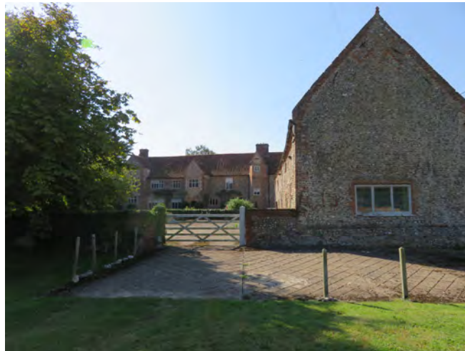
North elevation of Sharrington Hall Barn
