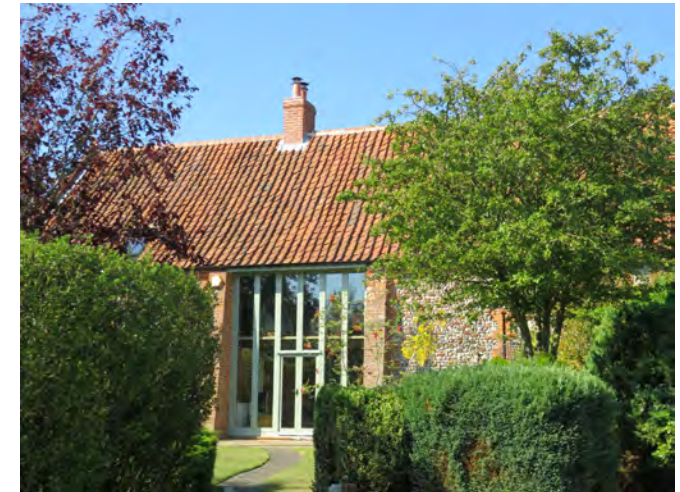
East elevation of Sharrington Hayloft converted barn showing glazing in barn door opening
