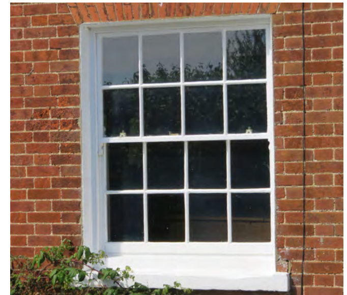
Detail of sash window from The Chequers
