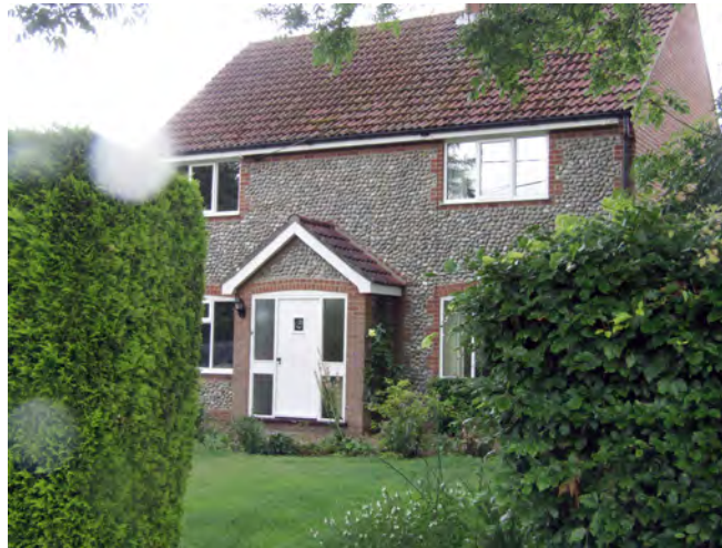
Modern house located on The Street
