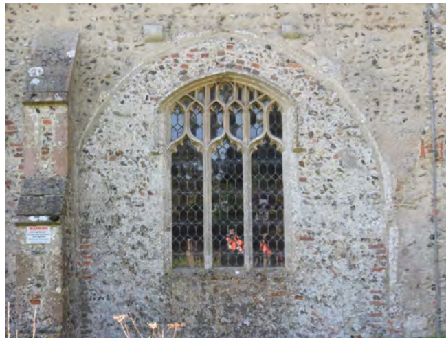
Window on the north elevation of All Saints' Church
