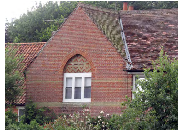
Detail of window on The Old Rectory
