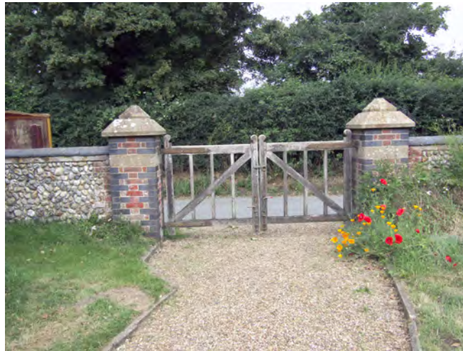
Cobble flint and red brick wall around the churchyard with attractive gate piers and timber gate
