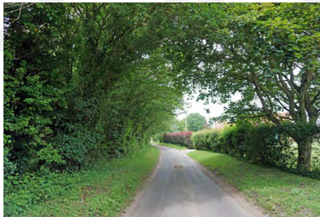
View of Brinton Road showing grassy verges on both sides
