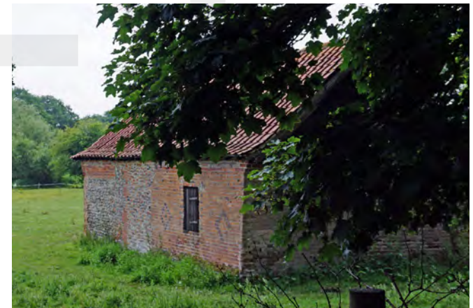
Farm building east of Kendles Farm complex with diapered brick pattern
