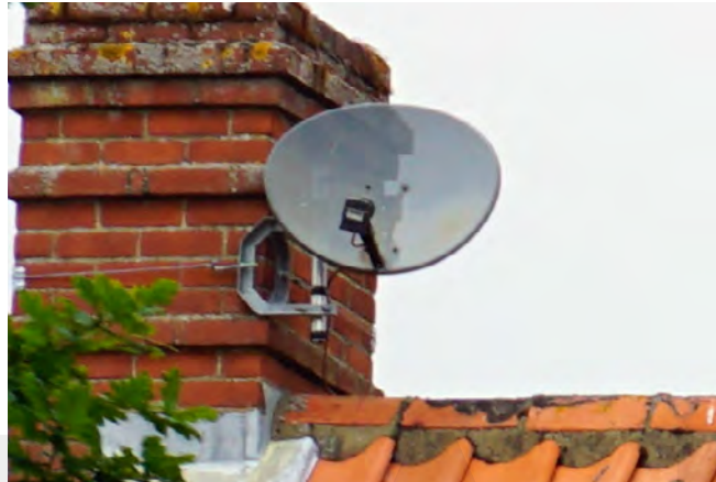
Visible satellite dish
