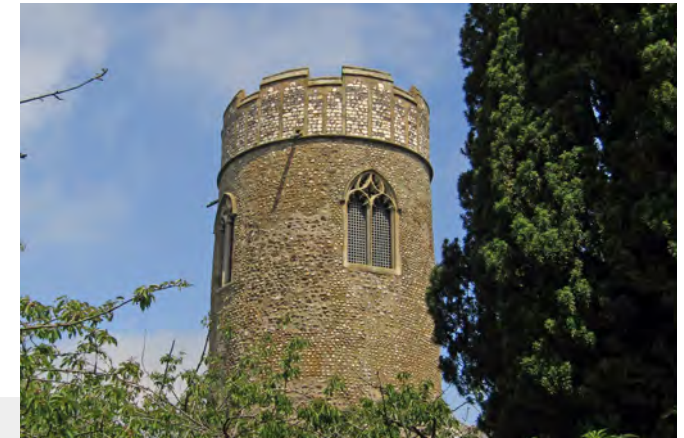
View of knapped flint trefoil pattern on upper part of church tower
