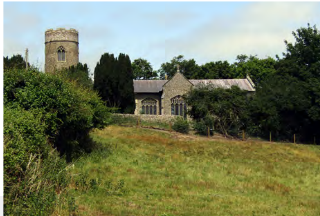
South elevation of the Church of St Mary
