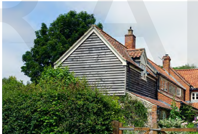
Modern weatherboarding on gable end of historic house
