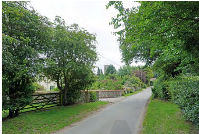
Showing the sensitive transition to the newly built red brick and flint wall beside the historic wall on properties east of Brinton Road
