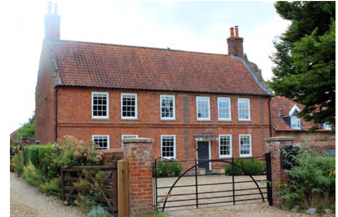
Thornage Grange on Letheringsett Road
