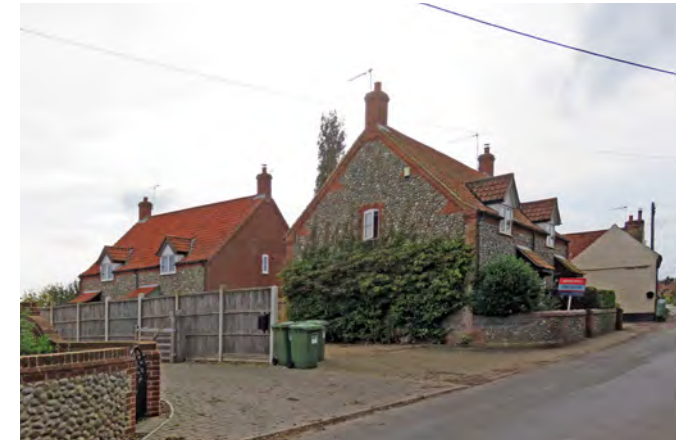
Modern semi-detached cottages on The Holt Road
