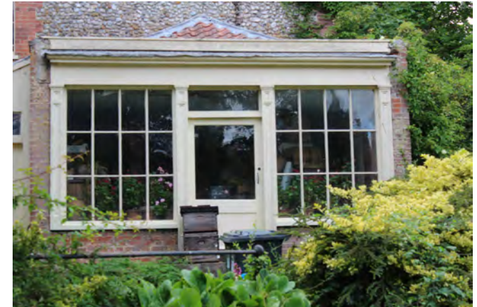
Converted nineteenth century shop front
