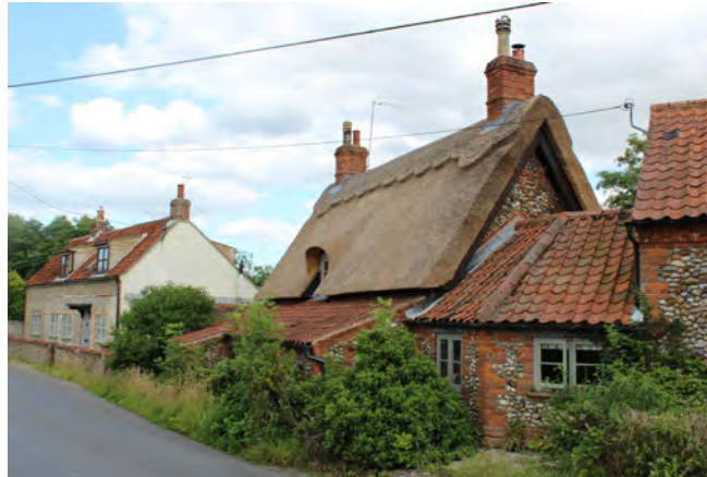
Bridge House Cottage at the south end of The Street
