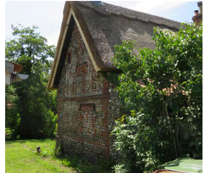
North gable end of the thatched house
