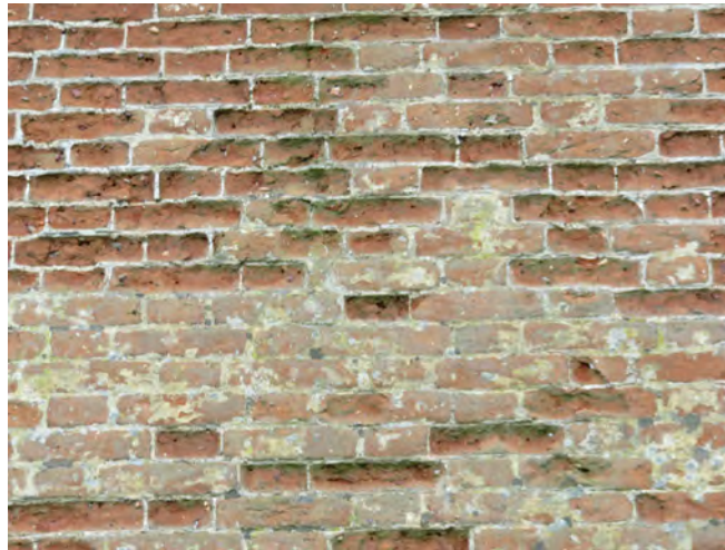
Brick delamination
