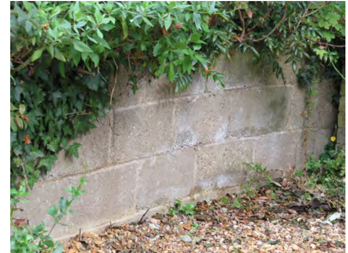
Example of a breezeblock wall
