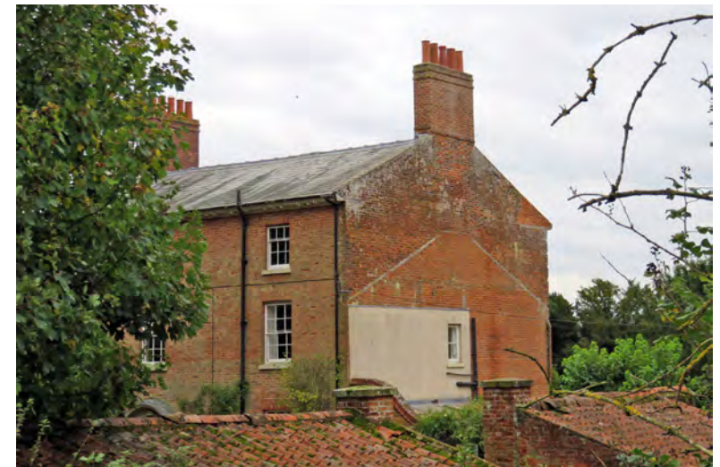
Rear elevation of The Old Rectory
