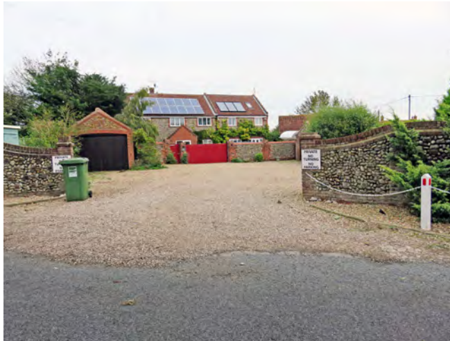
Very open access point, large no parking signs and poor road surfacing all detract from the character of the Conservation Area
