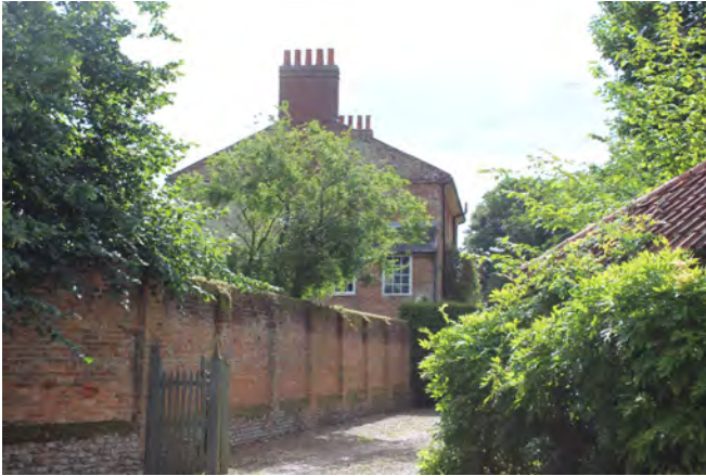
Tall and long stretch of wall at The Rectory
