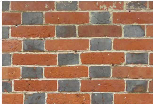
Flemish bond brick work
