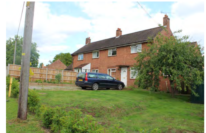
Modern semi-detached houses on The Street
