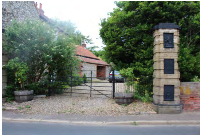
Gate pier containing Latin inscription and figurative castings of former brass and iron foundry on Holt Road
