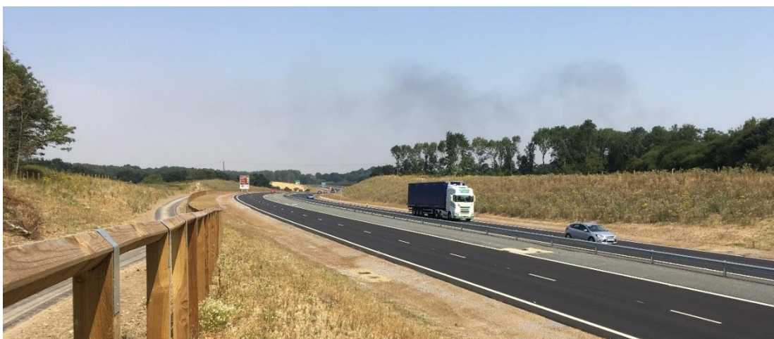
Photo of a newly created swale with over the edge drainage on Broadland Northway, Norwich, Norfolk (Image E Simpson @ NCC LLFA)
