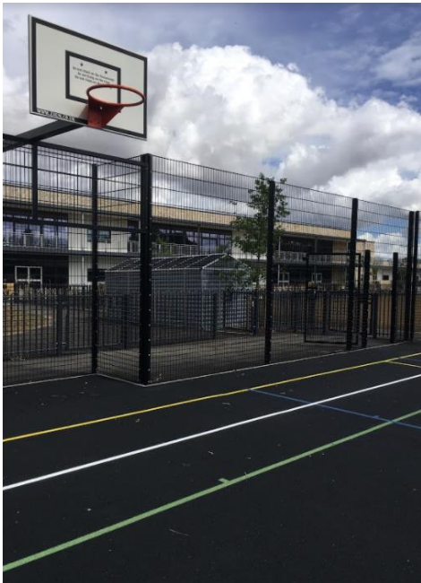
Photo of the use of permeable tarmac on a playground at the SEN School Old Buckingham, Norfolk (Image E Simpson @ NCC LLFA)
