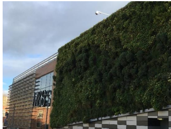
Photo of a green wall on a commercial building in an inner-city area, Norwich, Norfolk (Image E Simpson @ NCC LLFA)
