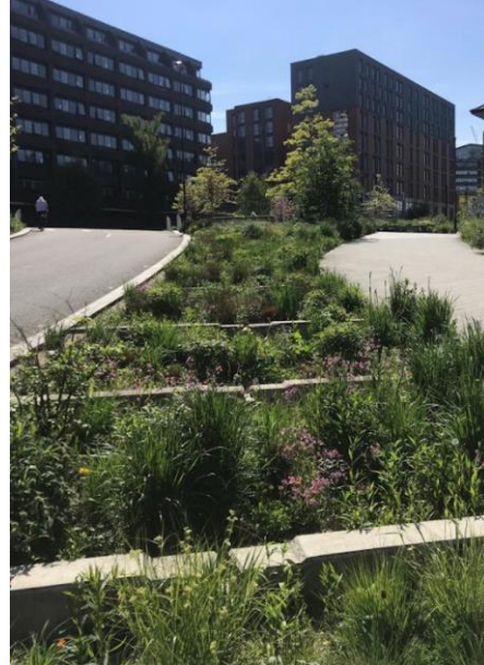
Photo showing example of retrofit SuDs: Planted under drained raingarden, over the edge drainage from the highway and paths. Sheffield Grey to Green Project.
