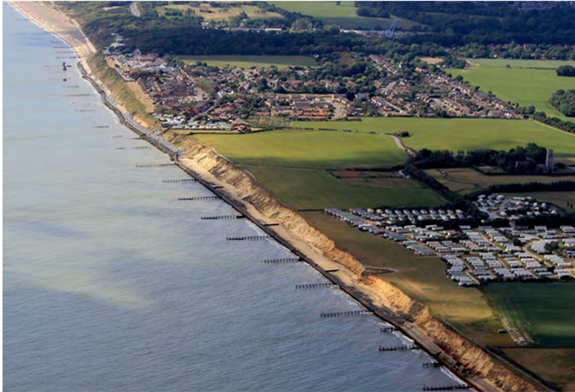
Aerial view of Corton showing cliffs, groynes and caravan parks
