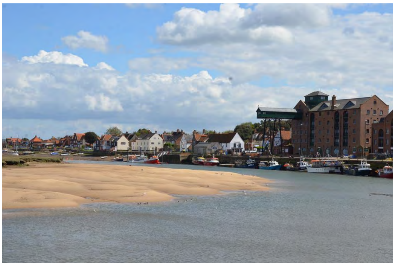
Wells-next-the-Sea harbour and historic granary building
