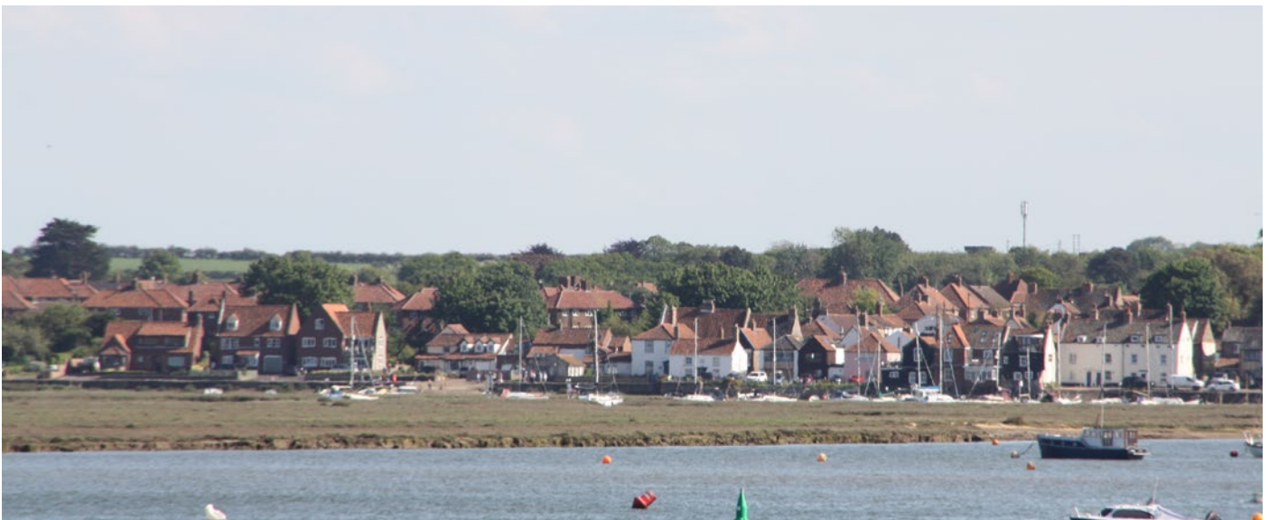
Figure 67: The average building height within the town is between 2-2.5 storeys. The subtle variation in the eaves and ridge levels create a harmonious roofline that is well integrated with the vegetation and countryside in the background.
