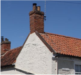
Gabled roof with red pantiles
