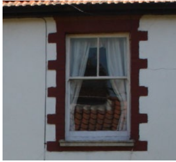
Sash window with brickwork
