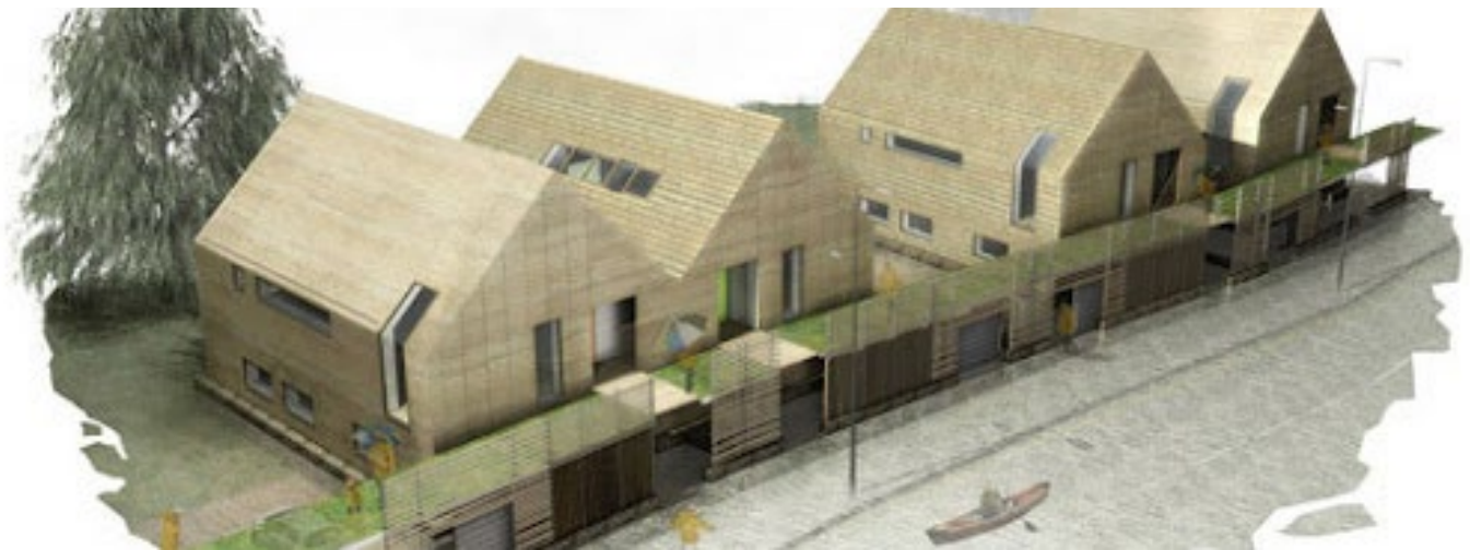
Figure 91: Example of adaptive architecture where living spaces are raised to respond to potential flooding. For most of the year, it serves as a typical house and only in a flood does it transform to allow an alternative 'turned around' living arrangement to be adopted. (Source: https://www.ice.org.uk/getattachment/media-and-policy/policy/facing-up-to-rising-sea-levels/Facing-Up-to-Rising-Sea-Levels-Document-Final.pdf.aspx ).
