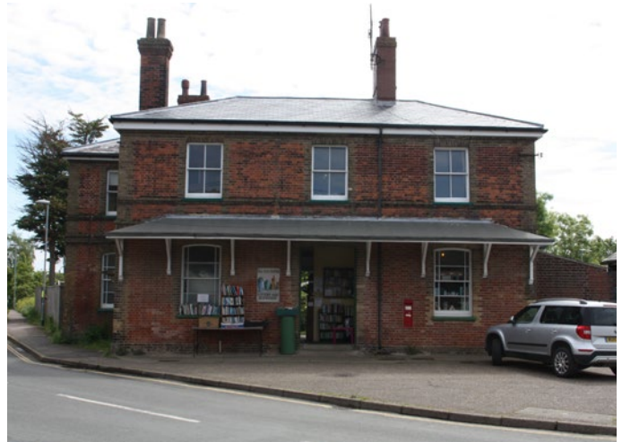
Figure 69: The old station, that is now used as pottery and bookshop, is a building of great historic significance with buffed red brick on the facade and sash windows which have been preserved over time.
