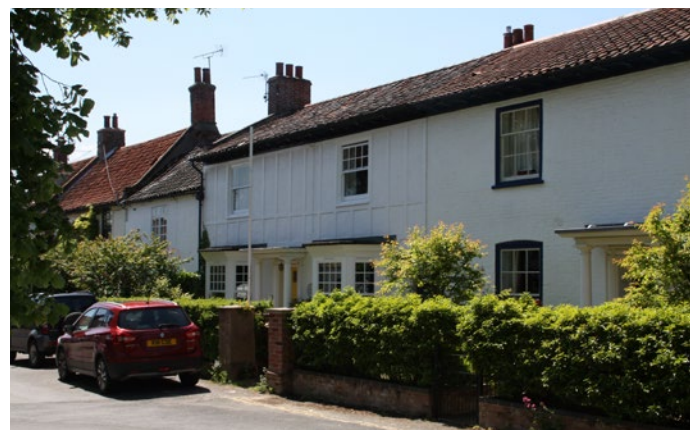
Figure 42: Local example of physical boundary treatment in the front gardens which also allows for clear views to the street ensuring a level of natural surveillance.
