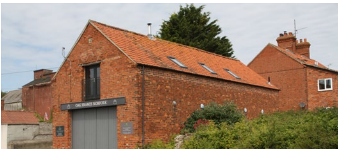
Figure 68: There are many industrial buildings in the town, mainly to the east, that sit well with the surrounding residential neighbourhoods by reflecting a similar style and massing (e.g. red bricks, gabled roofs).
