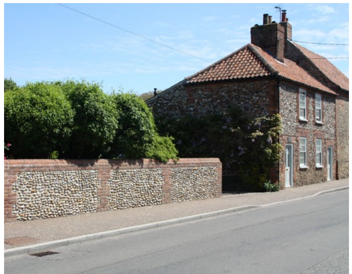
Figure 70: The use of flint with some brickwork on the building facades and the walls is a characteristic of the town and this can be found mainly within its historic core.
