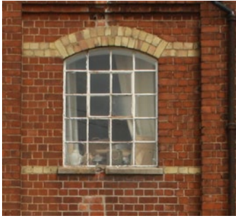
Timber painted window with yellow brickwork around
