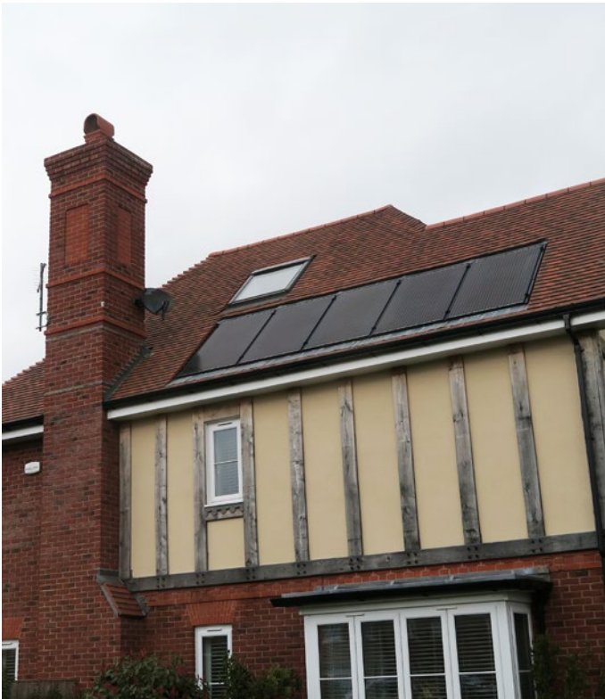
Figure 86: Integration of solar panels on the south-facing side of the roof of a new house in Lingfield, Surrey. The dark colour of the solar panels nicely matches with the dark brown tiles of the roof.
