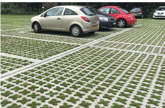
Figure 28: Examples of permeable sustainable materials that are durable and can manage surface water run-off. (Source: https://gridforce.co.uk/car-parks ).
