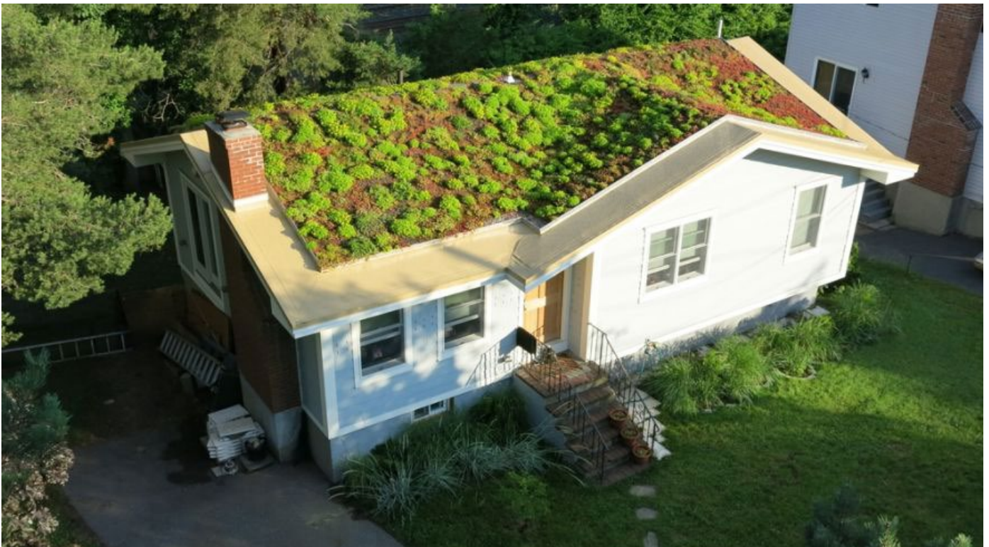
Figure 89: Green roof integrating the building with the surrounding landscape (Source: https://earlyexperts.net/green-roofing-a-house-advantages-and-costs/ ).
