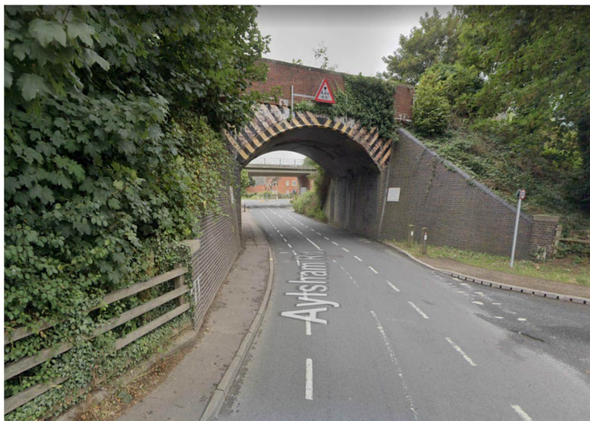
Figure 5-1 – Eastbound Road view on Aylsham Road at A149 underpass
