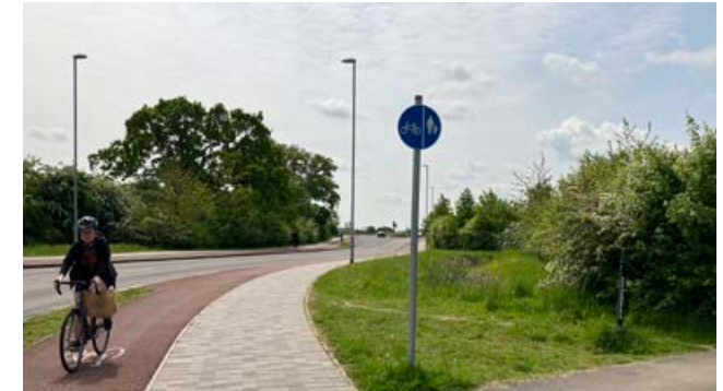
Figure 72; Example of development fronting a link road with footpath/cycleway, Eddington, Cambridge
