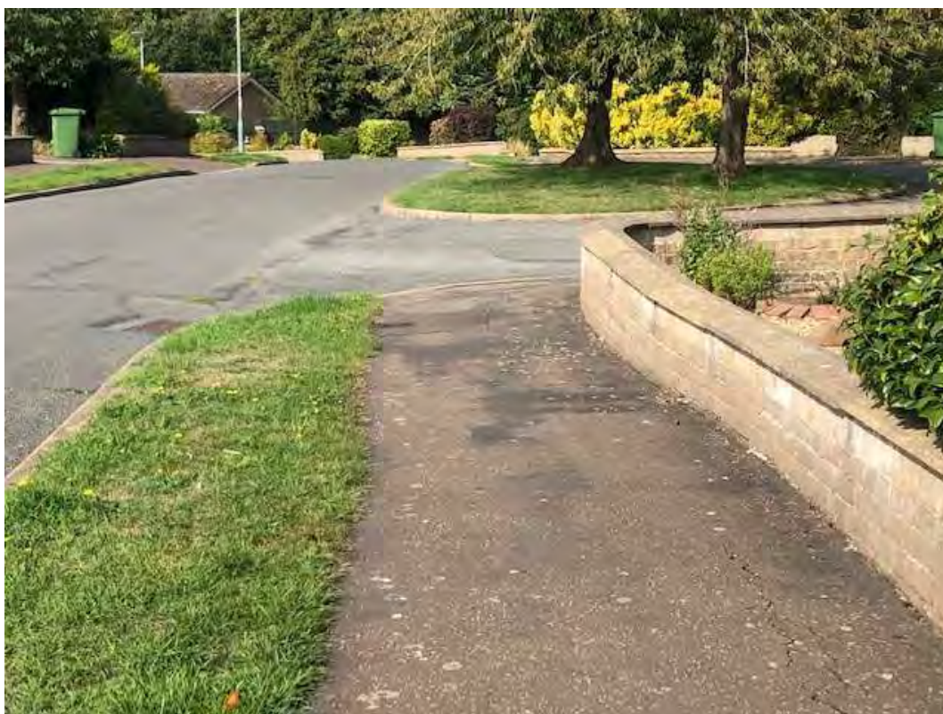
FIG 51 NORTHERN FOOTWAY OF BURNT HILLS – GOOD FOOTWAY PROVISION
