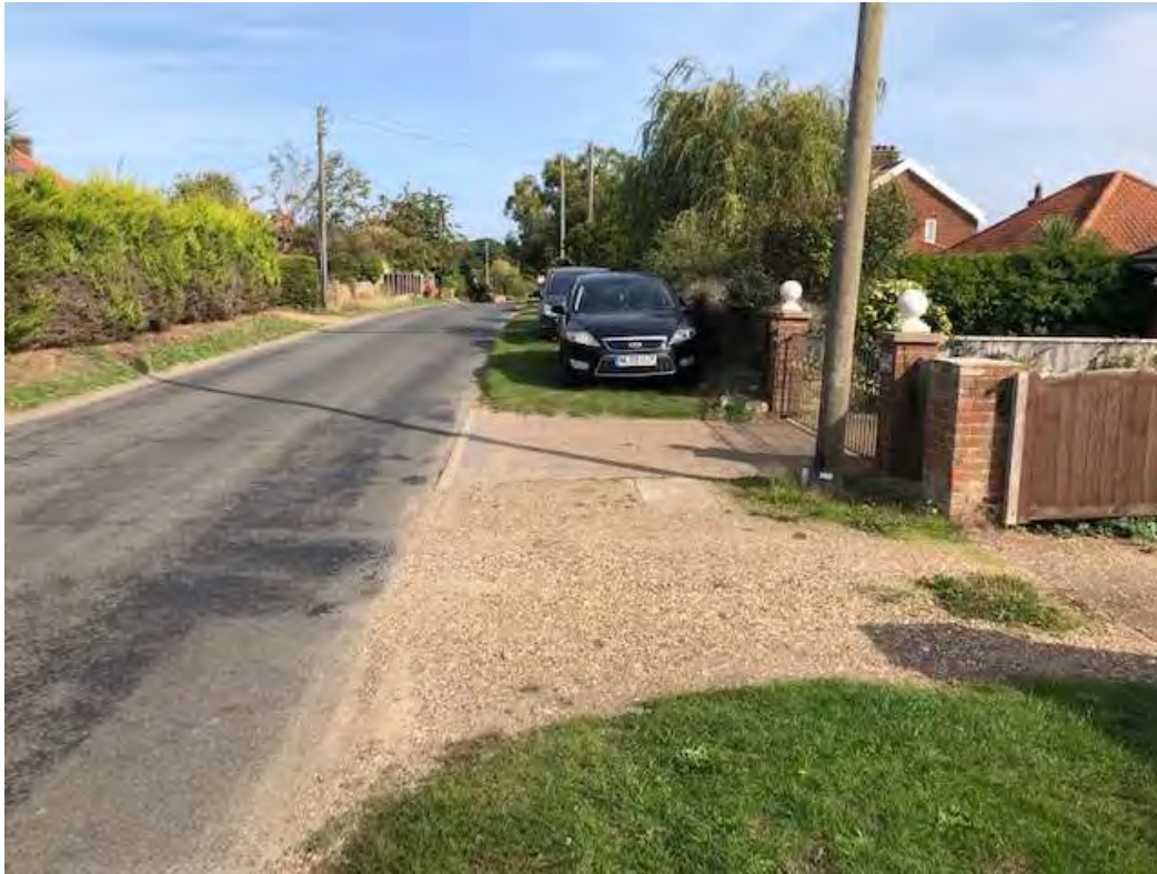
FIG 38 EASTERN VERGE ROUGHTON ROAD LOOKING NORTHWARDS WIDTH FOR NEW FWAY/CWAY.
