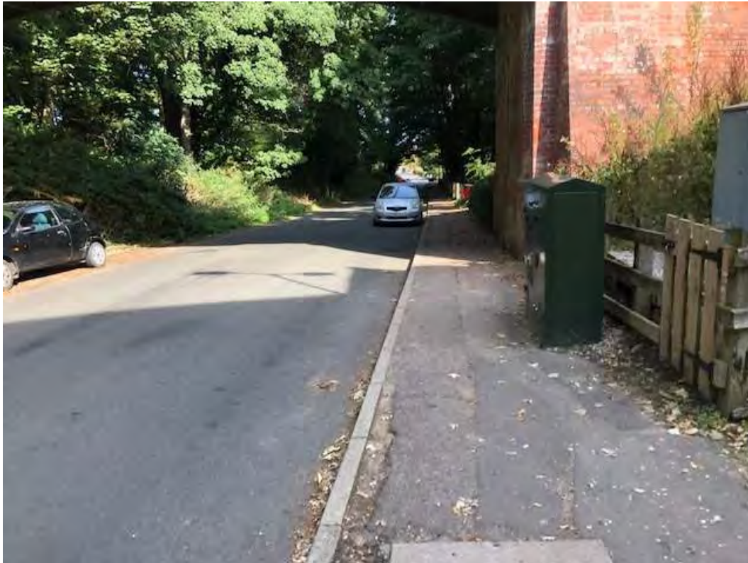
FIG 57 EASTERN FOOTWAY ROUGHTON ROAD UNDER NORWICH/CROMER RAILWAY LINE
