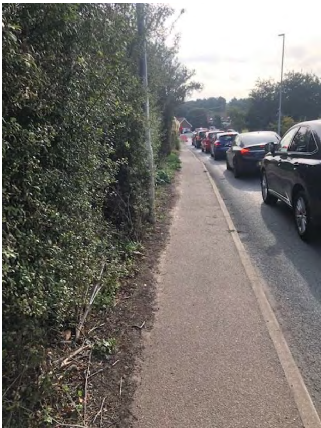
FIG 20 EASTERN FOOTWAY OF NORWICH ROAD LOOKING NORTHWARDS -RESTRICTED WIDTH
