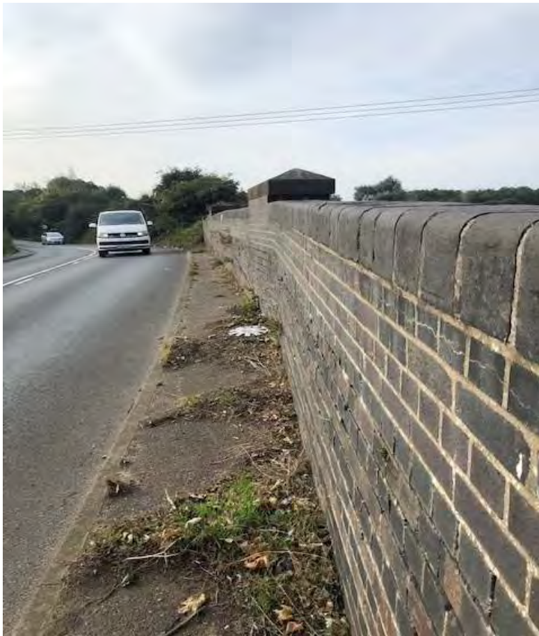
FIG 6 VIEW SOUTHWARDS ON OVERBRIDGE WESTERN VERGE- RESTRICTED WIDTH
