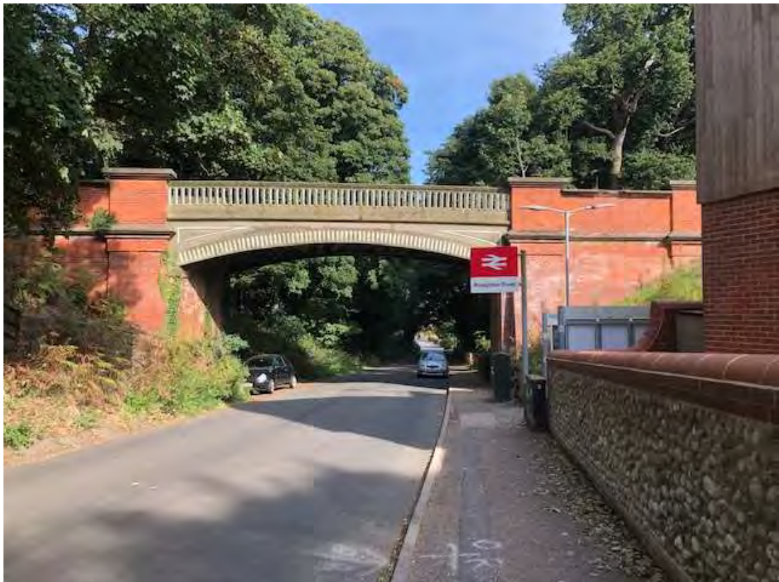
FIG ROUGHTON ROAD UNDRPASS
