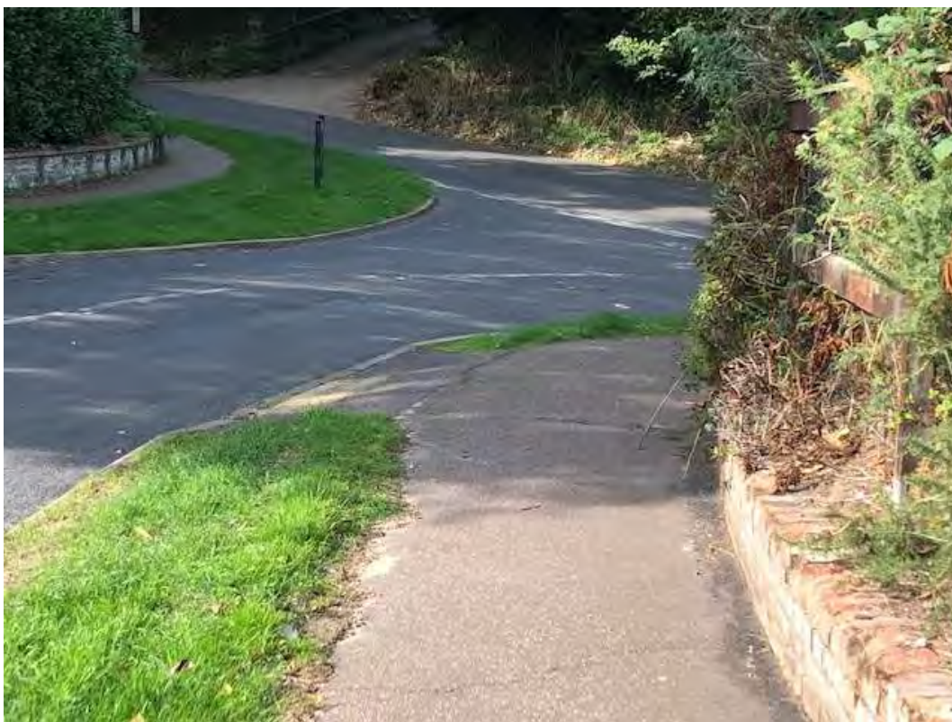
FIG 54 NORTHERN FOOTWAY OF BURNT MILLS JOINING ROUGHTON ROAD
