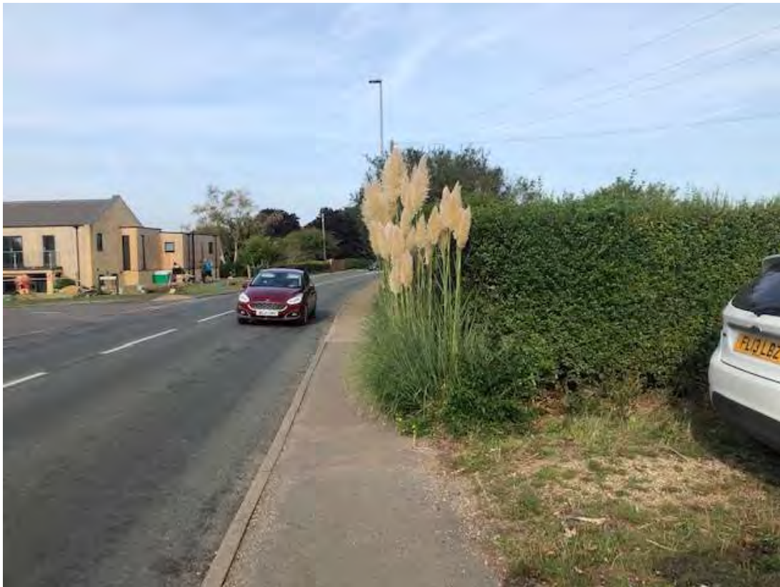
FIG 18 EASTERN FOOTWAY NORWICH ROAD LOOKING NORTHWARDS-OVERGROWN VEGETATION AND INSUFFICIENT WIDTH
