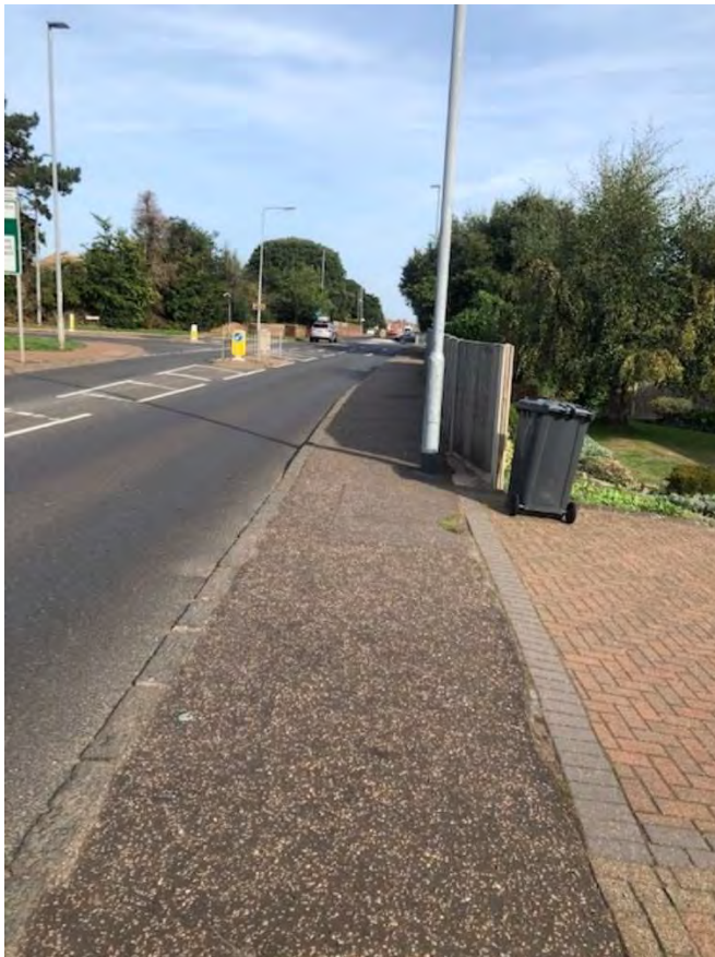
FIG 35 EASTERN FOOTWAY OF NORWICH ROAD VIEW ROUGHTON ROAD JUNCTION -POINT E
