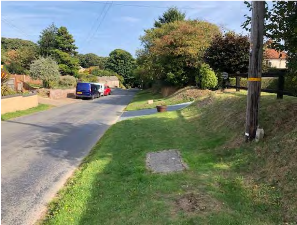
FIG 44 EASTERN VERGE ROUGHTON ROAD LOOKING NORTHWARDS WIDTH FOR NEW FWAY/CWAY
