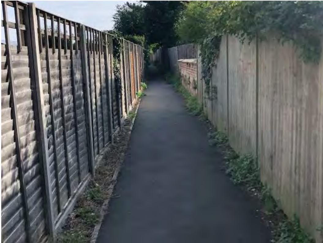
FIG 85 ROUGHTON ROAD TO NORWICH ROAD FOOTPATH LINK LOOKING EASTWARDS
