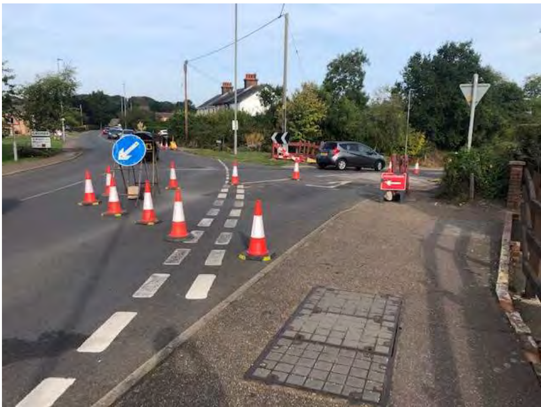
FIG 16 EASTERN FOOTWAY OF NORWICH ROAD CROSSING STATION ROAD
