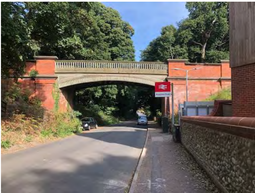
FIG 56 EASTERN FOOTWAY ROUGHTON ROAD NORTHWARDS TOWARDS ROUGHTON STATION.
