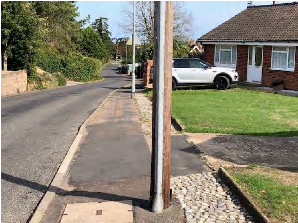
FIG 70 EASTERN FOOTWAY OF ROUGHTON ROAD NORTHWARDS TOWARDS NORWICH ROAD.
