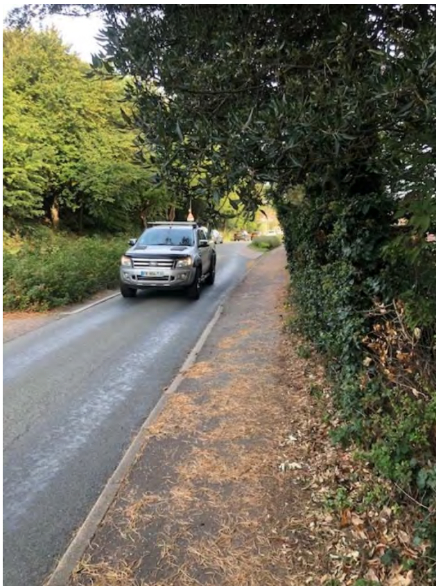
FIG 26 EASTERN FOOTWAY OF NORWICH ROAD ADJACENT TO TRAFFIC CALMING -RESTRICTED WIDTH AND OVERGROWN
