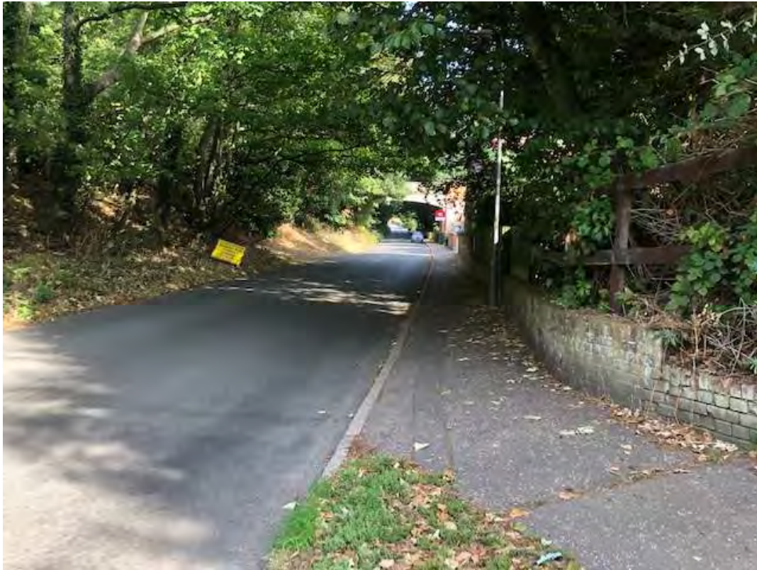
FIG 55 EASTERN FOOTWAY ROUGHTON ROAD FROM BURNT MILLS NORTHWARDS
