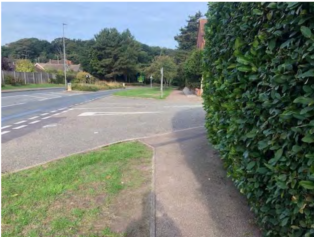
FIG 22 EASTERN FOOTWAY OF NORWICH ROAD CROSSING HIGHVIEW PARK -OVERGROWN
