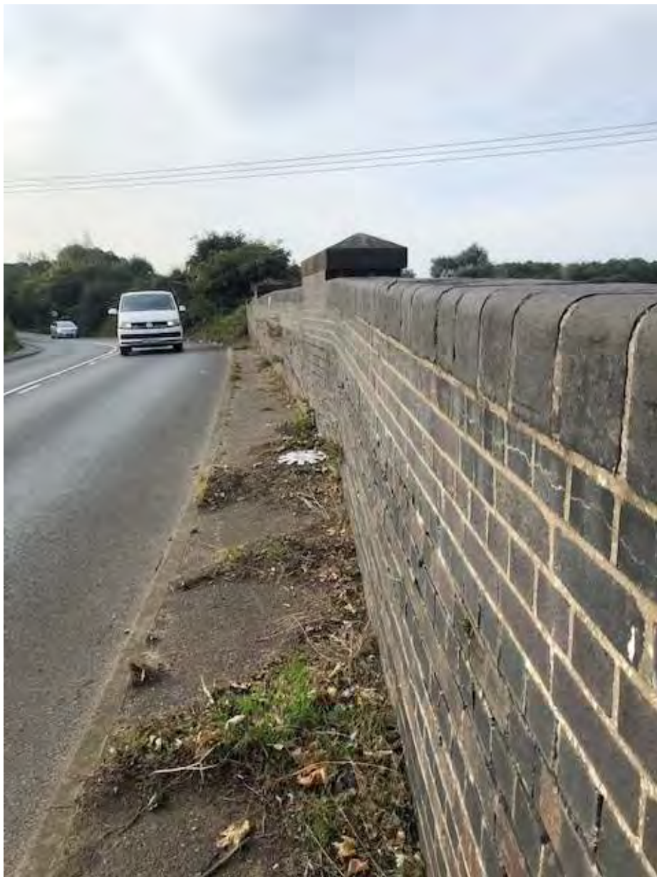
Figure showing western parapet of the Norwich Road Overbridge
