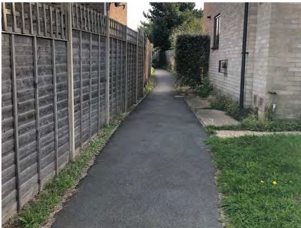
FIG 84 FOOTPATH LINK FROM ROUGHTON ROAD TO NORWICH ROAD LOOKING EASTWARDS
