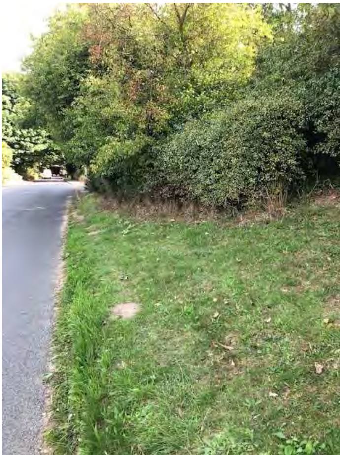
FIG 45 EASTERN VERGE ROUGHTON ROAD LOOKING NORTHWARDS TO BURNT MILLS JUNCTION EARTHWORKS REQUIRED AND PINCH POINT
