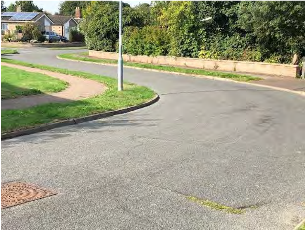
FIG 48 NORTHERN FOOTWAY OF BURNT HILLS
