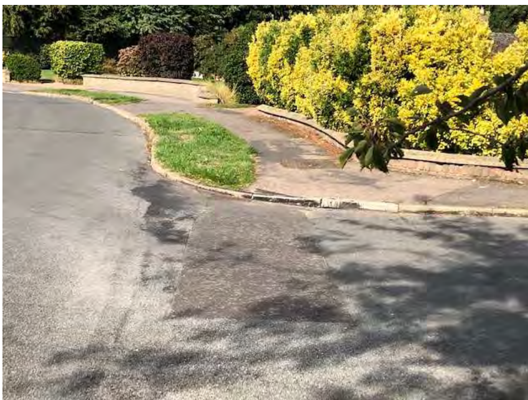
FIG 52 NORTHERN FOOTWAY OF BURNT HILLS -GOOD FOOTWAY PROVISION
