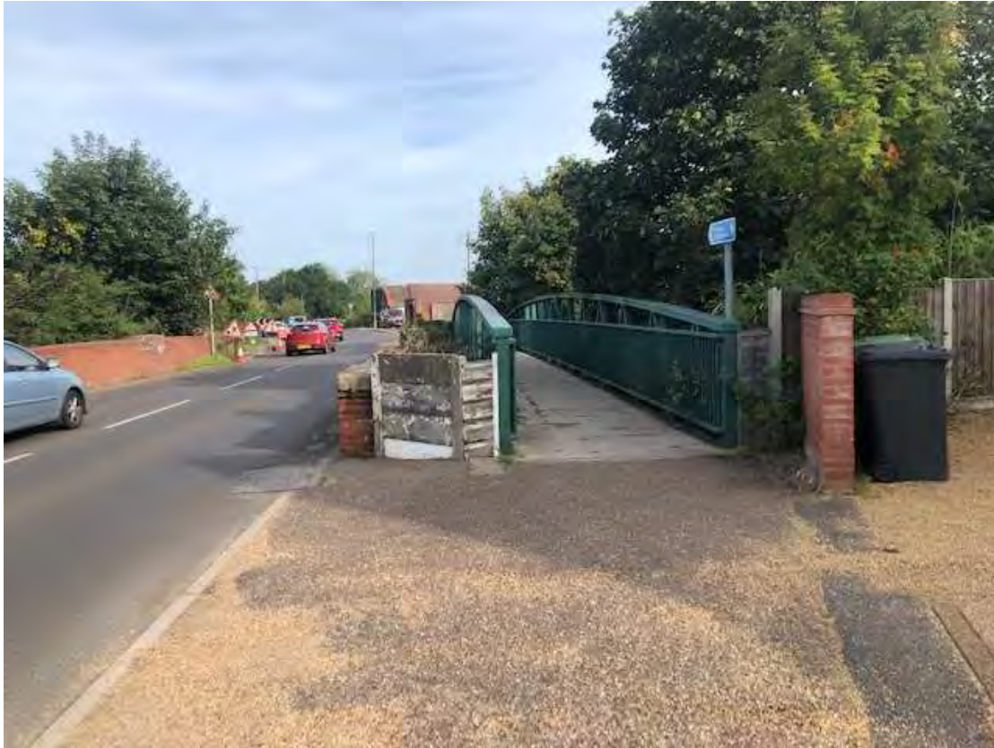
FIG 15 EASTERN FOOTWAY/CYCLEWAY BRIDGE OVER FORMER RAIL LINE
