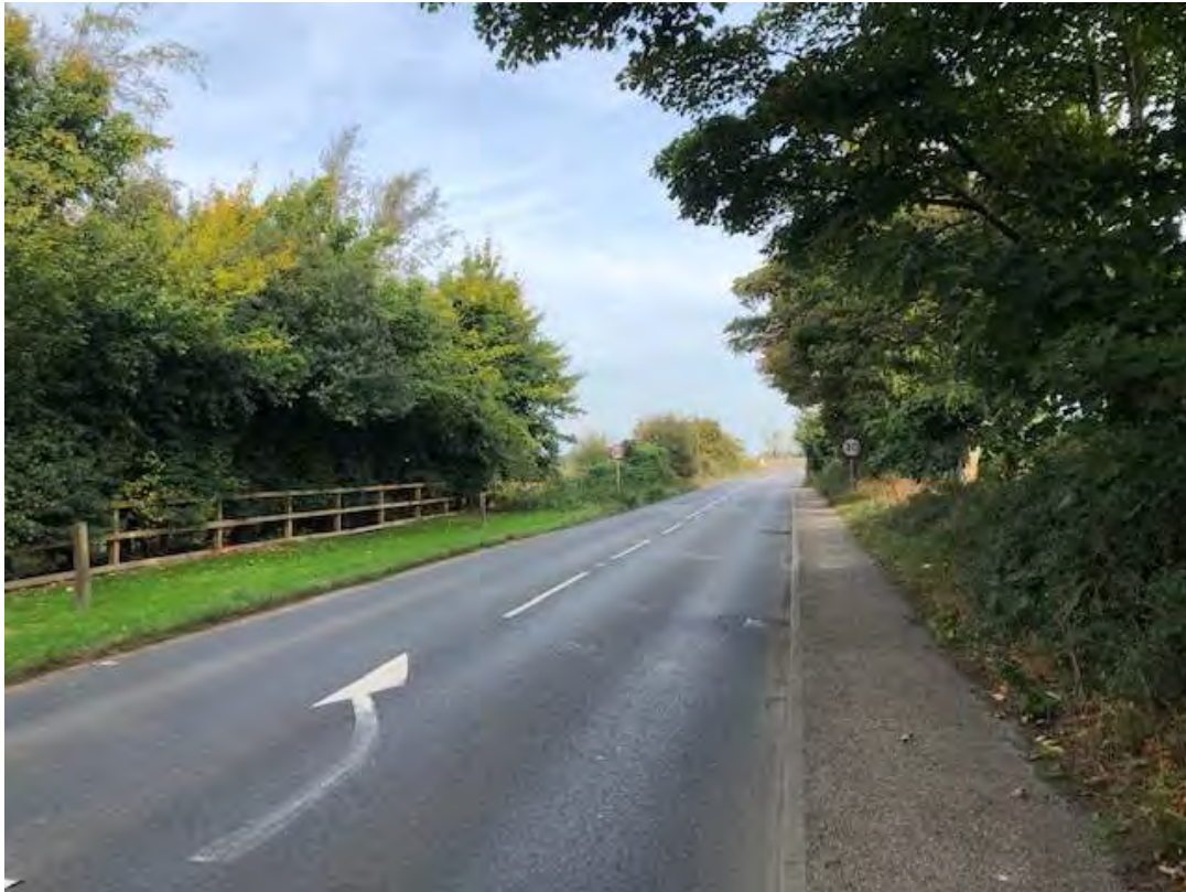
FIG 1 VIEW NORTHWARDS TOWARDS NORWICH ROAD OVERBRIDGE -RESTRICTED WIDTH BUT CAN BE IMPROVED.
