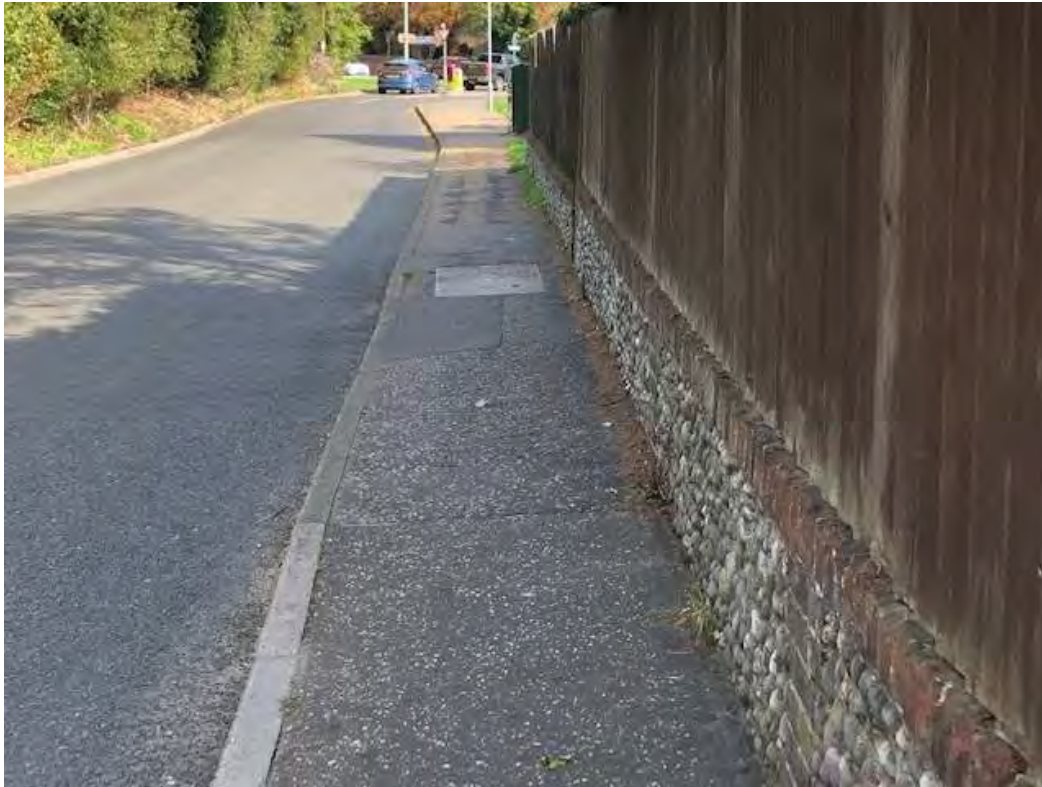
FIG 73 EASTERN FOOTWAY OF ROUGHTON ROAD NORTHWARD TOWARDS NORWICH ROAD
