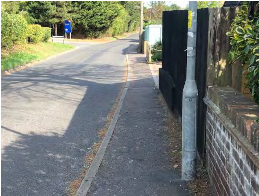
FIG 72 EASTERN FOOTWAY OF ROUGHTON ROAD NORTHWARDS RESTRICTED WIDTH ALTHOUGH SPACE TO WIDEN CROMER HOSPITAL SIDE
