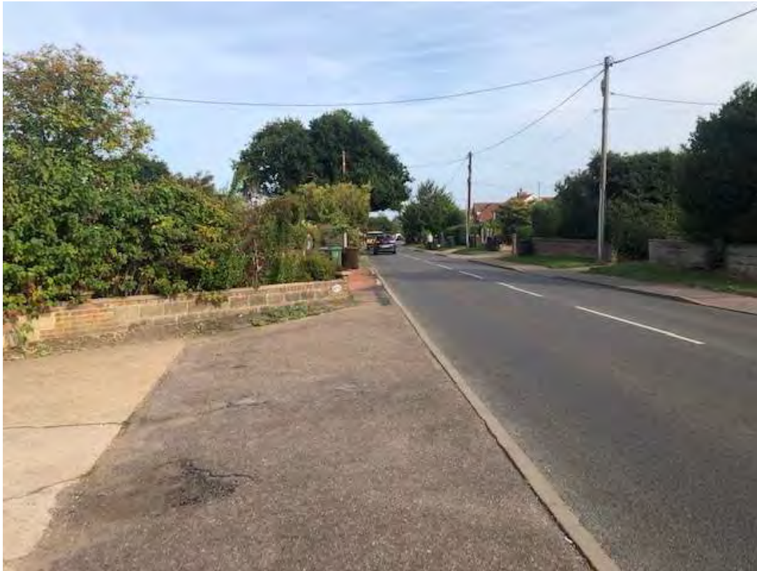
FIG 11 WESTERN VERGE OF NORWICH ROAD LOOKING NORTHWARDS-NO AVAILABLE WIDTH
