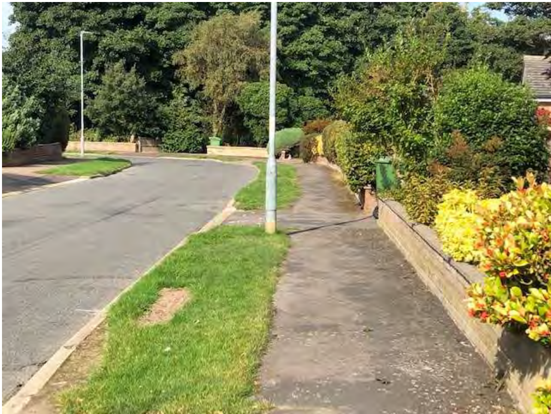
FIG 47 NORTHERN FOOTWAY OF BURNT HILLS. -GOOD FOOTWAY PROVISION
