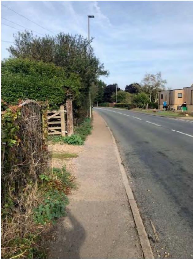
FIG19 EASTERN FOOTWAY OF NORWICH ROAD LOOKING SOUTHWARDS -RESTRICTED WIDTH
