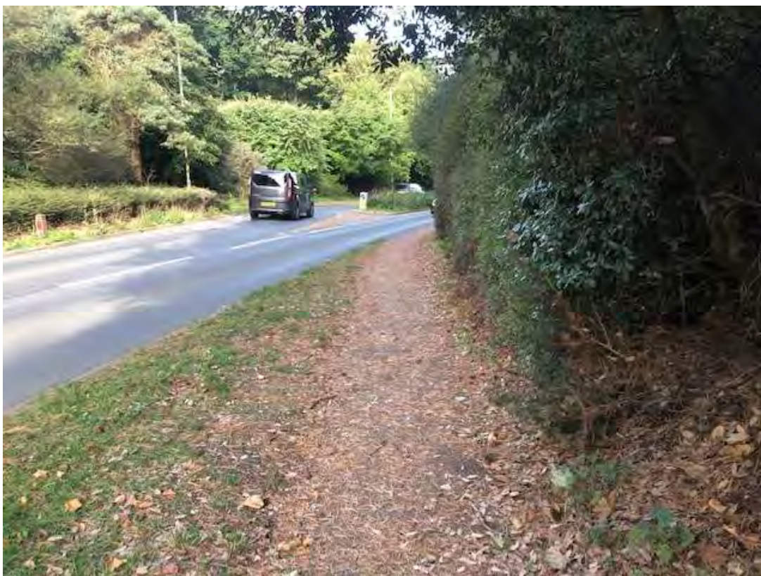
FIG 24 EASTERN FOOTWAY OF NORWICH ROAD LOOKING TOWARDS CHICCANE TRAFFIC CALMING - OVERGROWN RESTRICTING WIDTH
