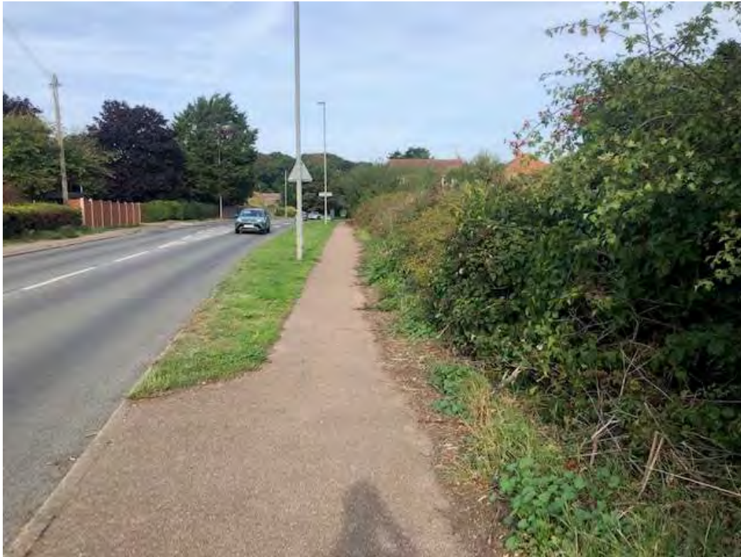
FIG 21 EASTERN FOOTWAY OF NORWICH ROAD LOOKING NORTHWARDS TOWARDS HIGHVIEW PARK-FOOTWAY OVERGROWN WITH VEGETATION RESTRICTING WIDTH
