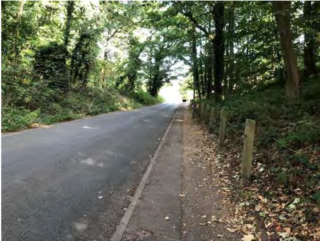
FIG 59 EASTERN FOOTWAY ROUGHTON ROAD NORTHWARDS BROWNSHILL
