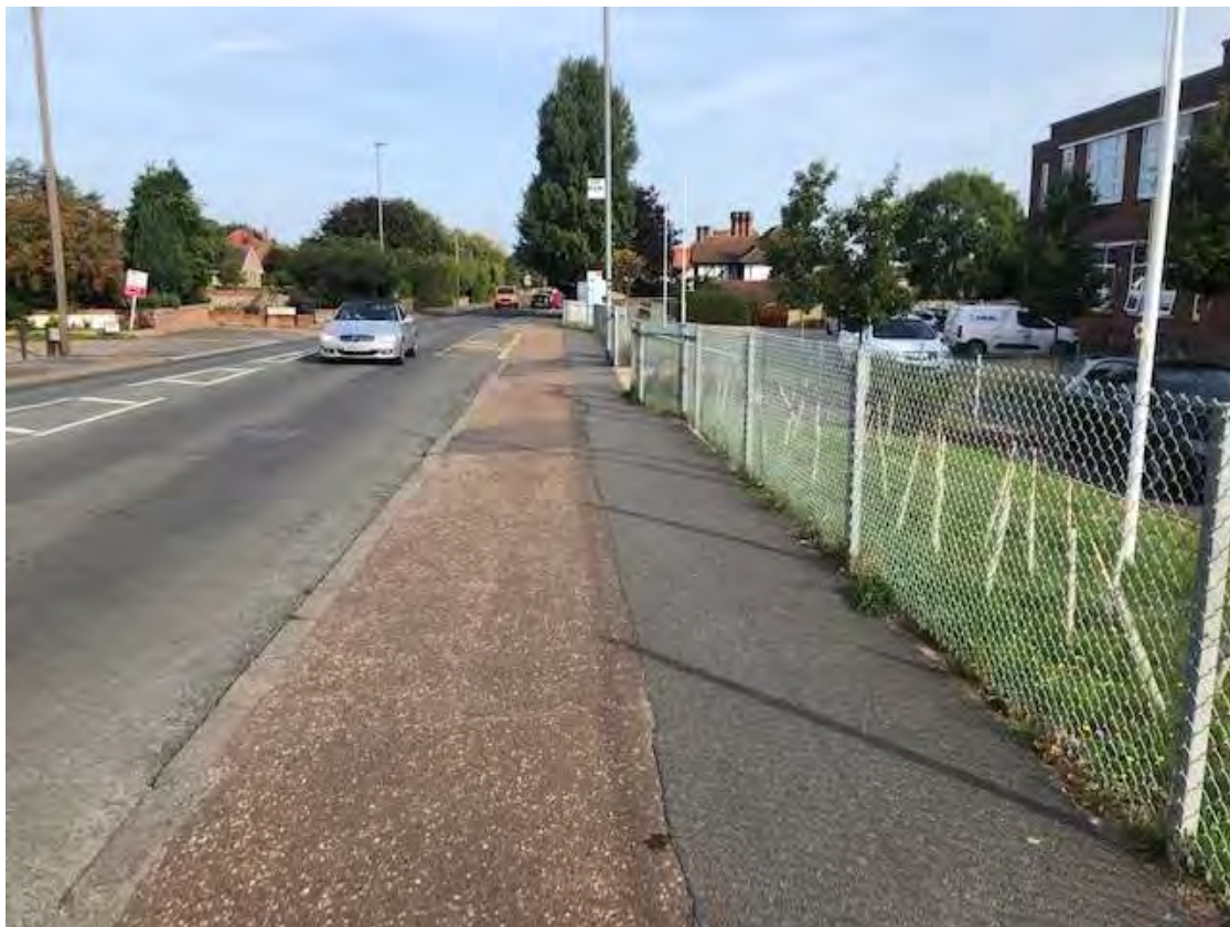
FIG 32 EASTERN FOOTWAY OF NORWICH ROAD AT CROMER ACADEMY ENTRANCE
