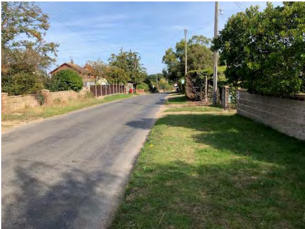
FIG 39 EASTERN VERGE ROUGHTON ROAD LOOKING NORTHWARDS WIDTH FOR NEW FWAY/CWAY
