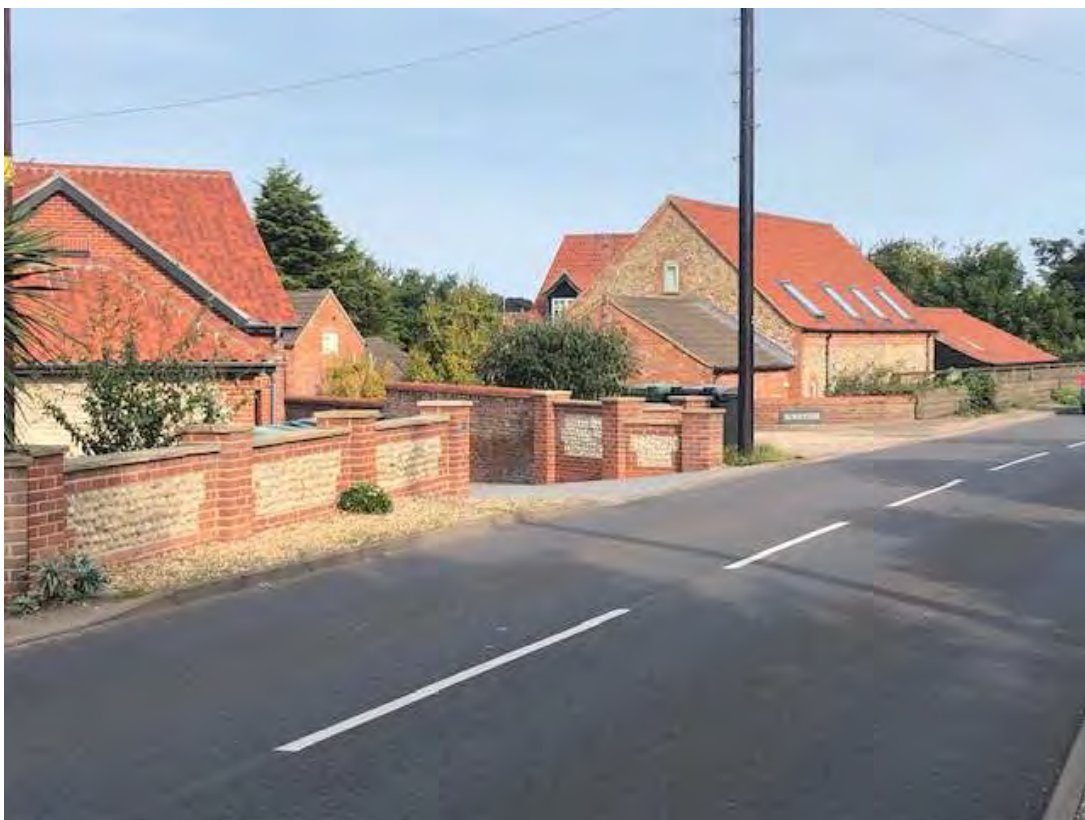
FIG12 WESTERN VERGE OF NORWCH ROAD LOOKING NORTHWARDS -RESTRICTED WIDTH
