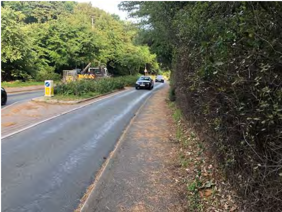
FIG 25 EASTERN FOOTWAY OF NORWICH ROAD ADJACENT TO TRAFFIC CALMING -OVERGROWN
