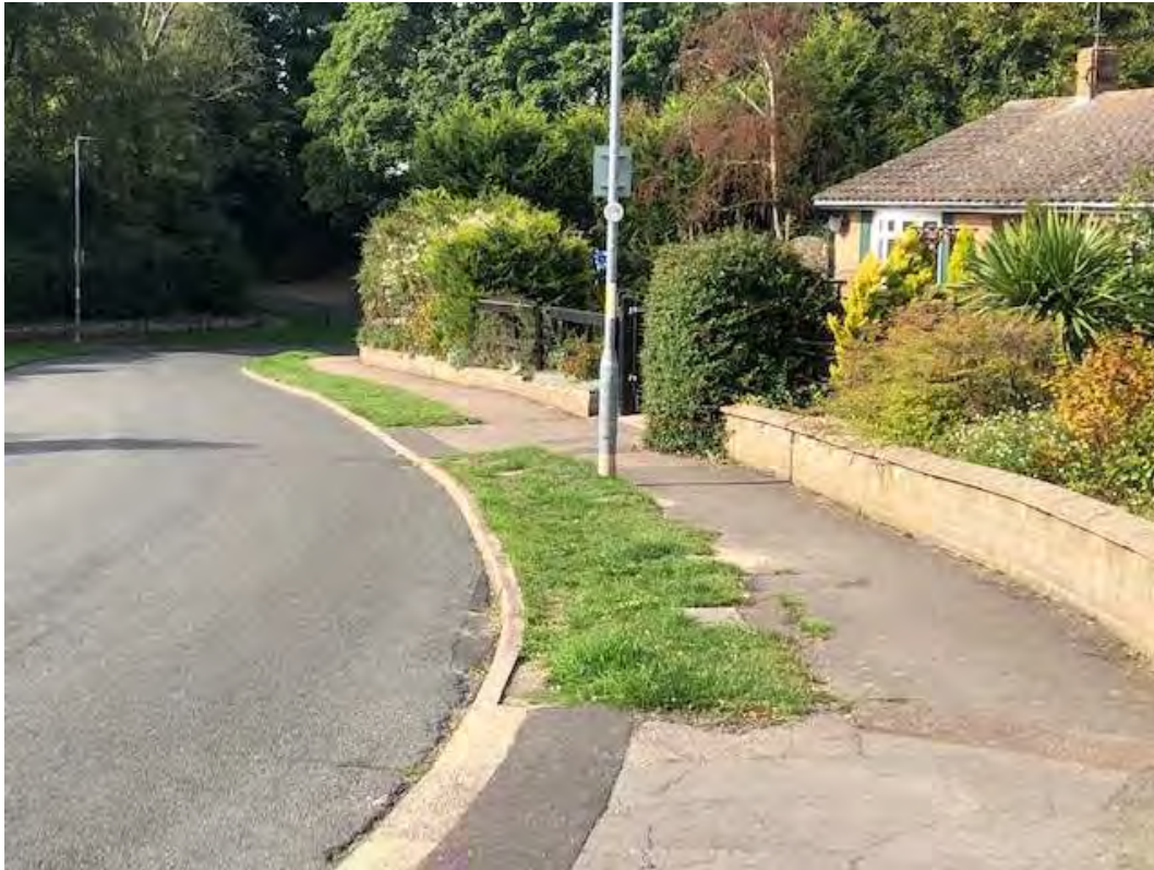
FIG 53 NORTHERN FOOTWAY OF BURNT HILLS GOOD FOOTWAY PROVISION
